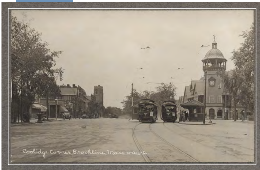
Coolidge Corner, Brookline, 1915.
