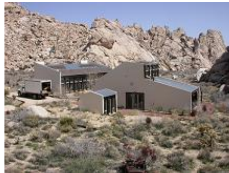
The Sybil and Al A. Allanson Center and Library consist of residence and laboratory buildings located in Granite Cove.
