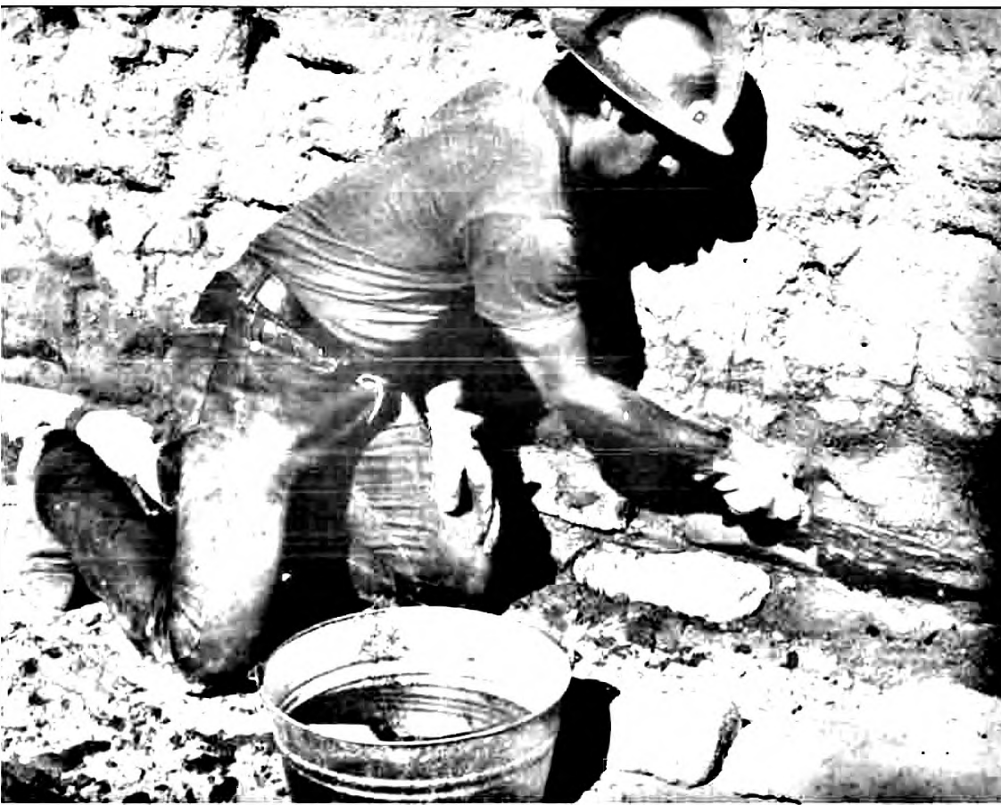
Caving—the hollowing out of an adobe wall just above grade—may be caused by standing rainwater, rainwater splash-up from the ground, or by salts deposited in the adobe by moisture evaporation. This adobe wall is being patched in the traditional manner with adobe mud.
