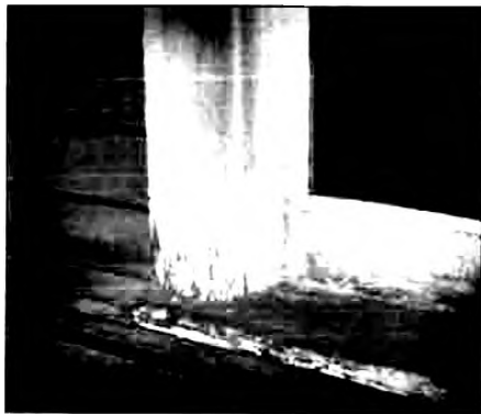
Deterioration of poorly maintained windows usually begins on horizontal surfaces where water collects. Problem areas on this sill are clearly indicated by paint failure due to moisture.
