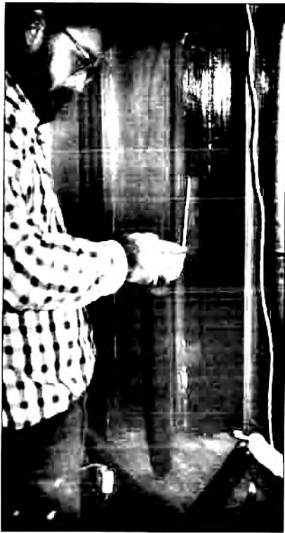
Maintaining a historic window may include work as basic as replacing a sash cord.
