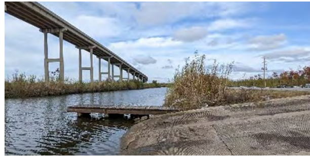
Gibbstown Bridge access site. NPS photo.
