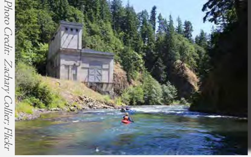
PacifiCorp Powerhouse seen from the river
