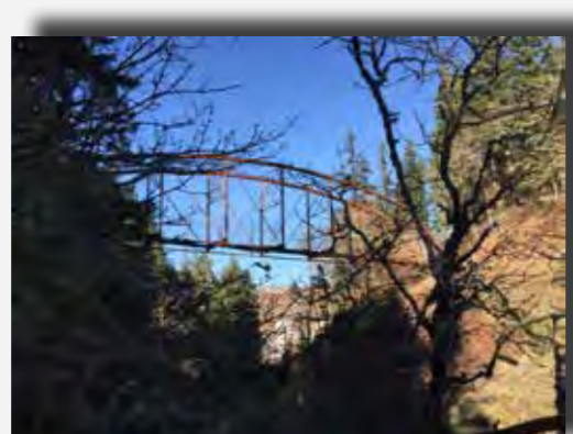
View of the bridge from the river
