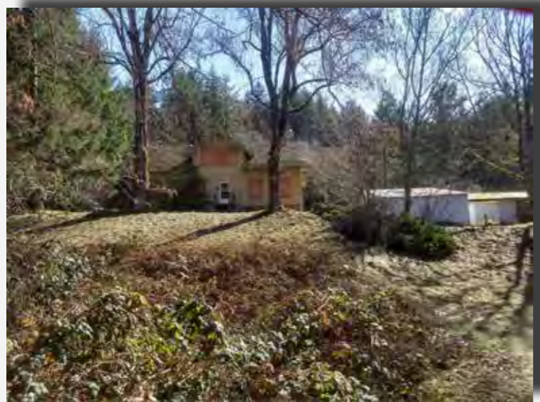
PacifiCorp building currently at the site
