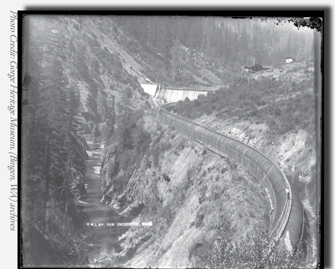
Aerial view looking upstream along Condit Dam penstock flume pipe
