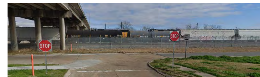
Below Enterprise Blvd, at South Railroad Avenue
