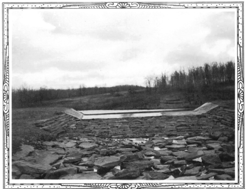
Alleg.4 Pro.F - Palmer Pond Auxillary spillway - apron con- creted. Stones below aprong to prevent wash. Taken 10/4/37 by I. S. Bowlby - Film T No.3
