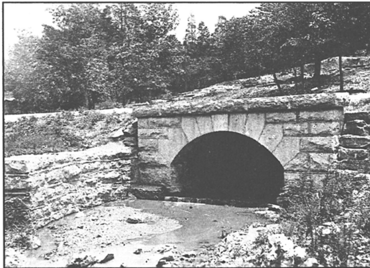
Figure 25. Stone culvert and headwall, intersection of Jay's Mill Road and Alexander Bridge Road
