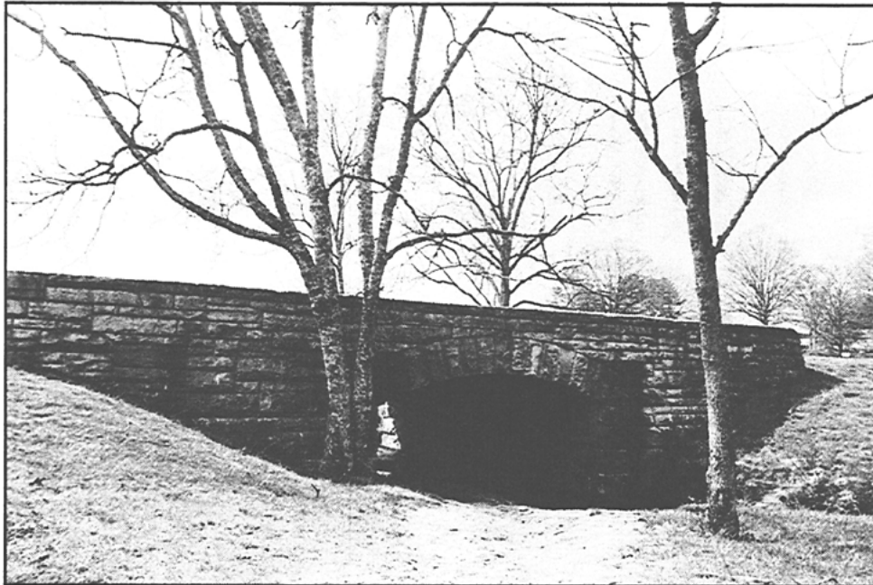
Figure 38. Stone bridge, U.S. Highway 27/Lafayette Road
