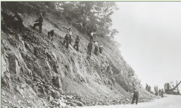
CCC workers build erosion controls along Skyline Drive. NPS, BELOW—NPS / ED KNEPLEY
