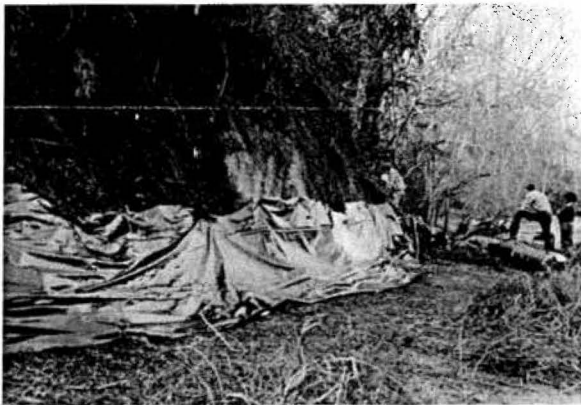
Figure 2. Installation of underliner
