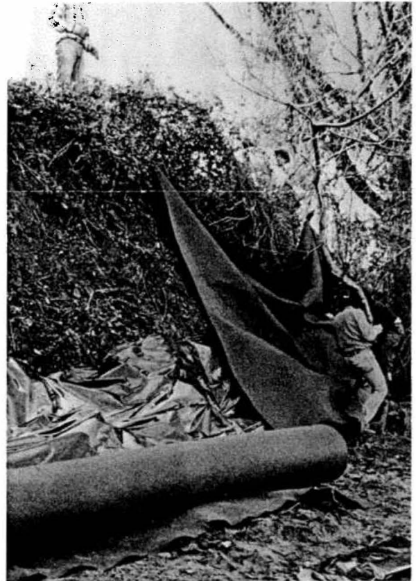
Figure 3. Installing filter fabric
