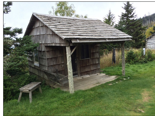
Employee Quarters Single Room Cabin
