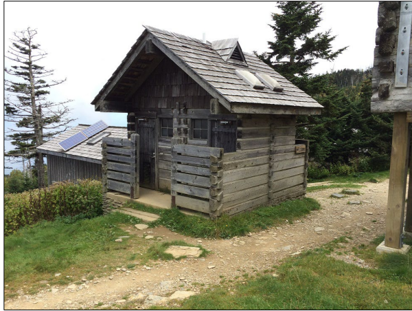
Flush Toilet for Guests and Employees
