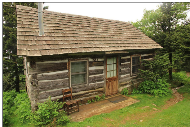
Employee Quarters, Shower and Laundry Building
