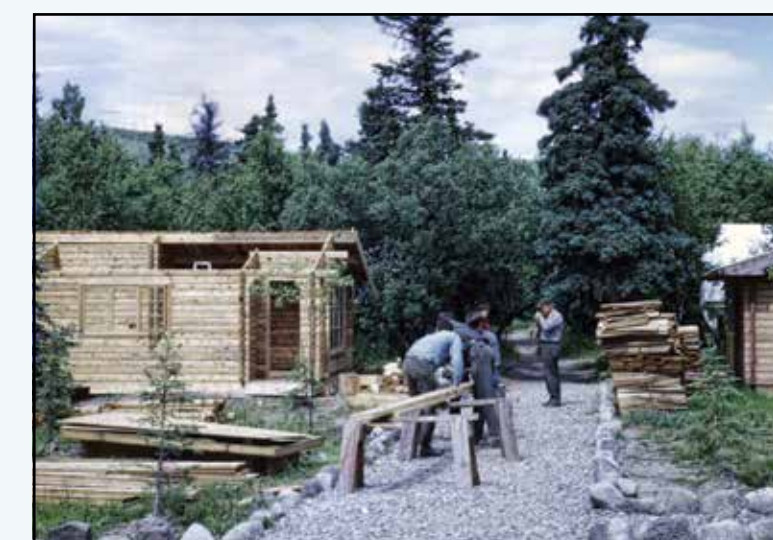
NPS constructing Pan Abode housing in 1962. NPS Photo.
