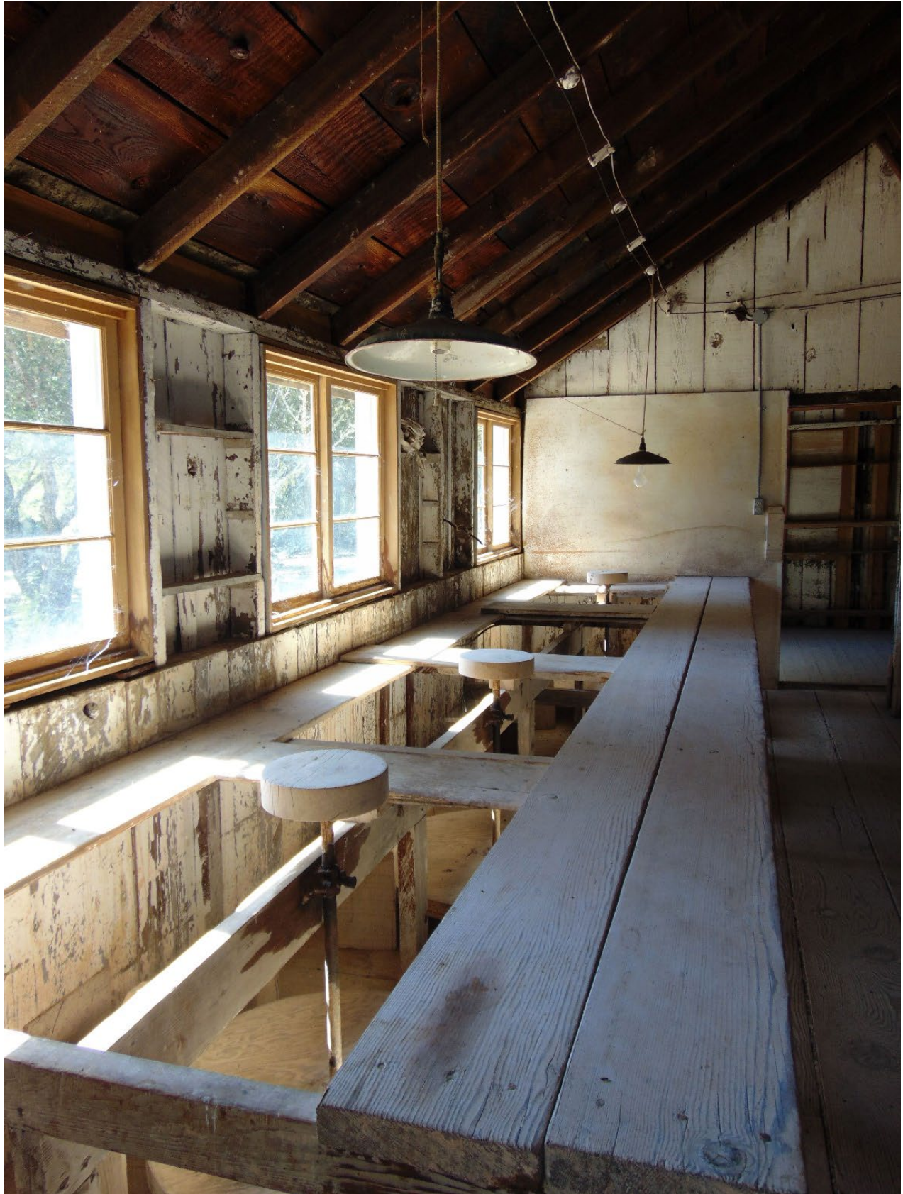
Photo 4: Barn interior, south studio, facing west. Photographed on September 25, 2018 by Ari Green.
