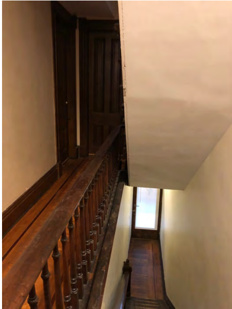
Second Floor and First Floor Hallways
