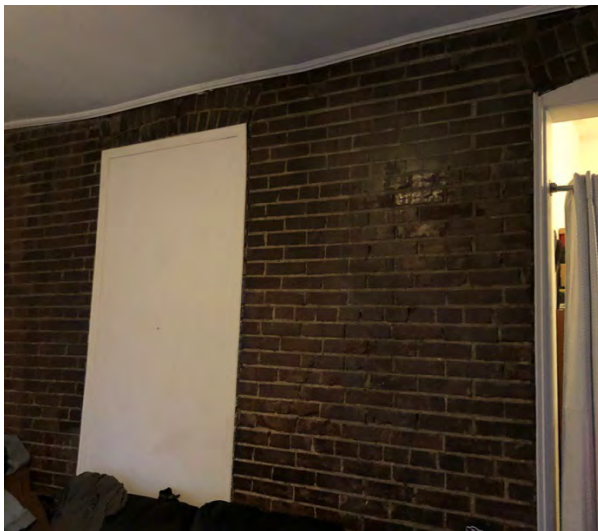
Exterior Brick Wall in Studio, Original to 1892-1905 Addition
