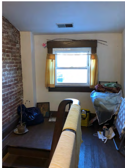
Third Floor Hallway
