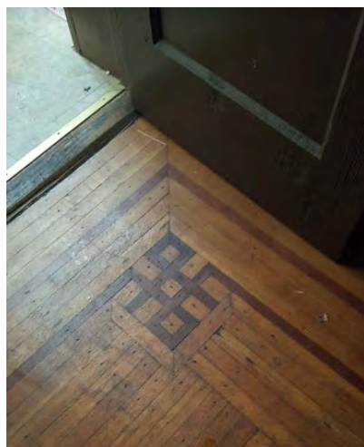
Detailed Inlay on First Floor
