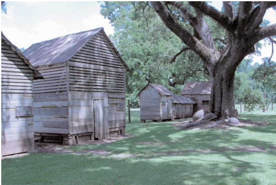
Fig. 1. Outbuildings at Oakland Plantation, part of Cane River Creole National Historical Park, located in the Bermuda Community south of Natchitoches, Louisiana. Many of these buildings date back to the nineteenth century, and their existence today is a reflection of the physical completeness of the site. Numerous outbuildings at Oakland Plantation are clad with wood siding that has weathered over time. All images by Sarah Jackson.
