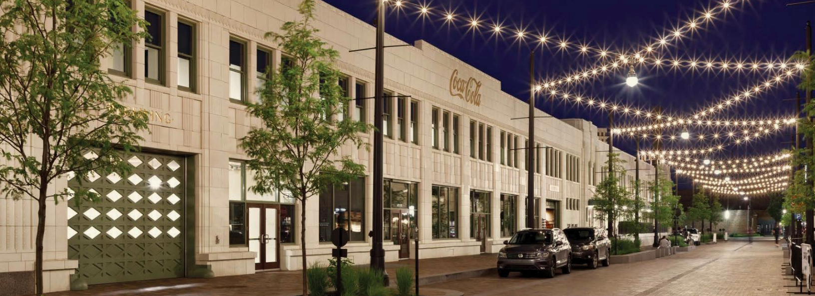
Coca-Cola Bottling Plant, Shipping Department after rehabilitation. Photo: Susan Fleck
