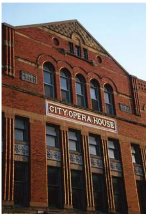
The City Opera House, (photo: NPS project file)
