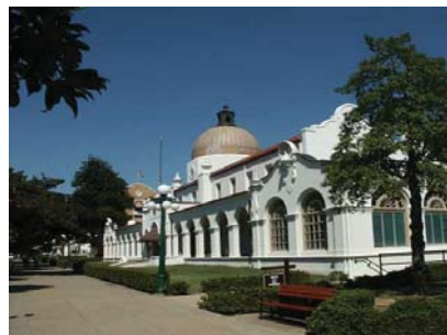
Quapaw Bathhouse, Hot Springs National Park, Arkansas, a certified rehabilitation project. (photo: National Park Service)
