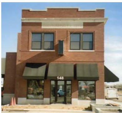
S.D. Robinett Building (photo: NPS project file)
