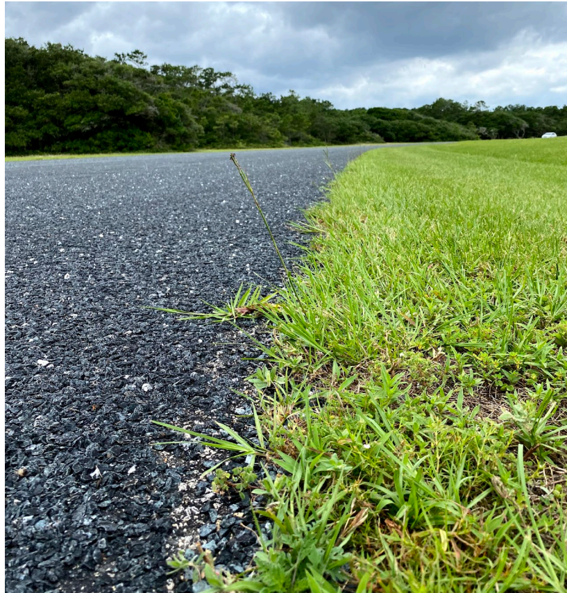
Figure 15: Typical Example of Weeds at Roadway Edge Causing Shuttle Disengagements Source: U.S. DOT Volpe Center
