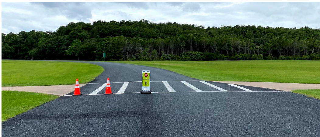
Figure 21: Cones and Signage Placed at High-Traffic Pedestrian Crossing Source: U.S. DOT Volpe Center
