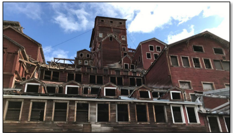
Picture of the Kennecott Mill Building
