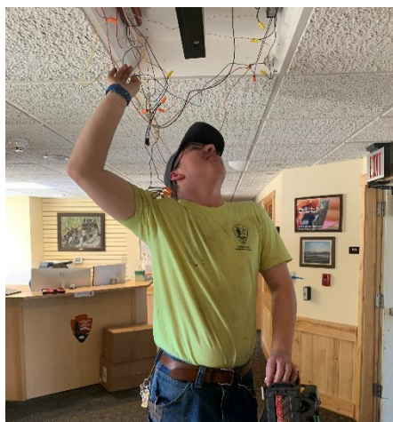
< Thomas Abraham replaces fluorescent light bulbs with energy-efficient bulbs at the Headquarters building. NPS
