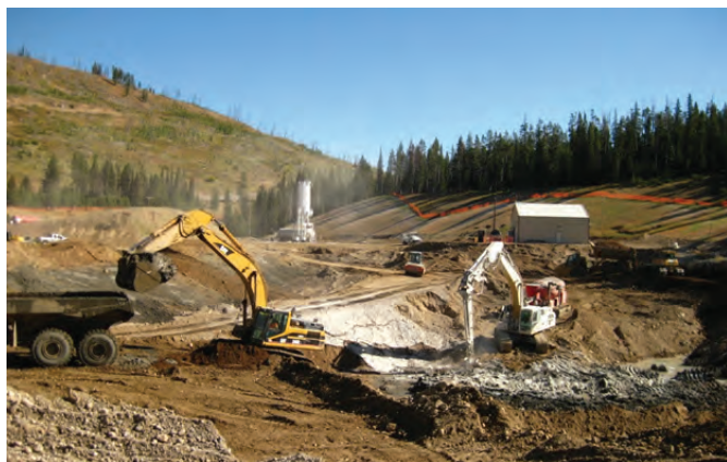
Lime mixing and excavation of tailings in 2012.
