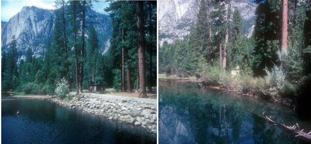
Figure 14: Before (left) and after (right) riverbank restoration through riprap removal and revegetation at the former Lower Rivers Campground. Riparian vegetation thrives on the riverbank.
