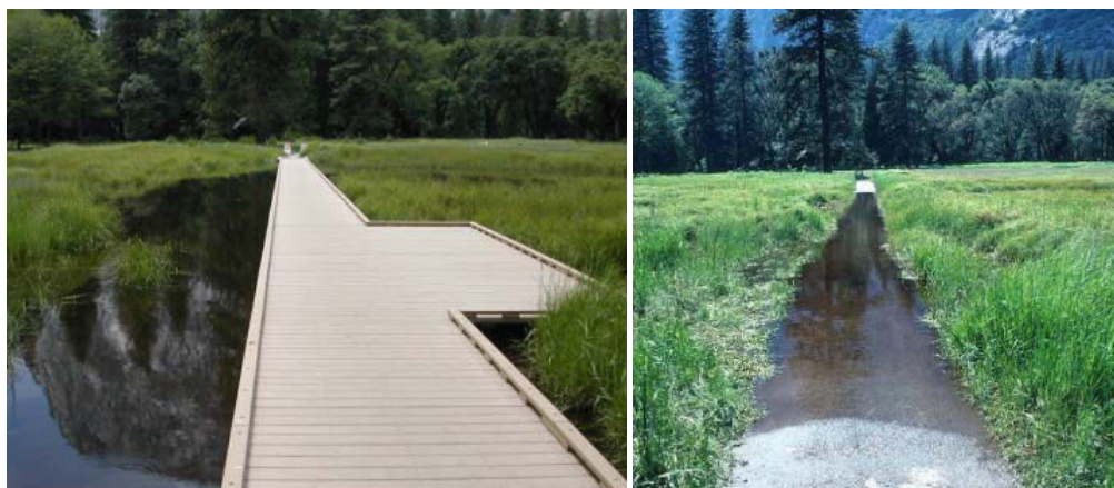
Figure 17: Trails through frequently inundated wet meadows, such as in cook's meadow pre-restoration (left), cause peripher vegetation trampling and soil compaction and make access difficult. A boardwalk installed in 2005 allows for visitor access into the meadow environment and protects the meadow soils and hydrology.
