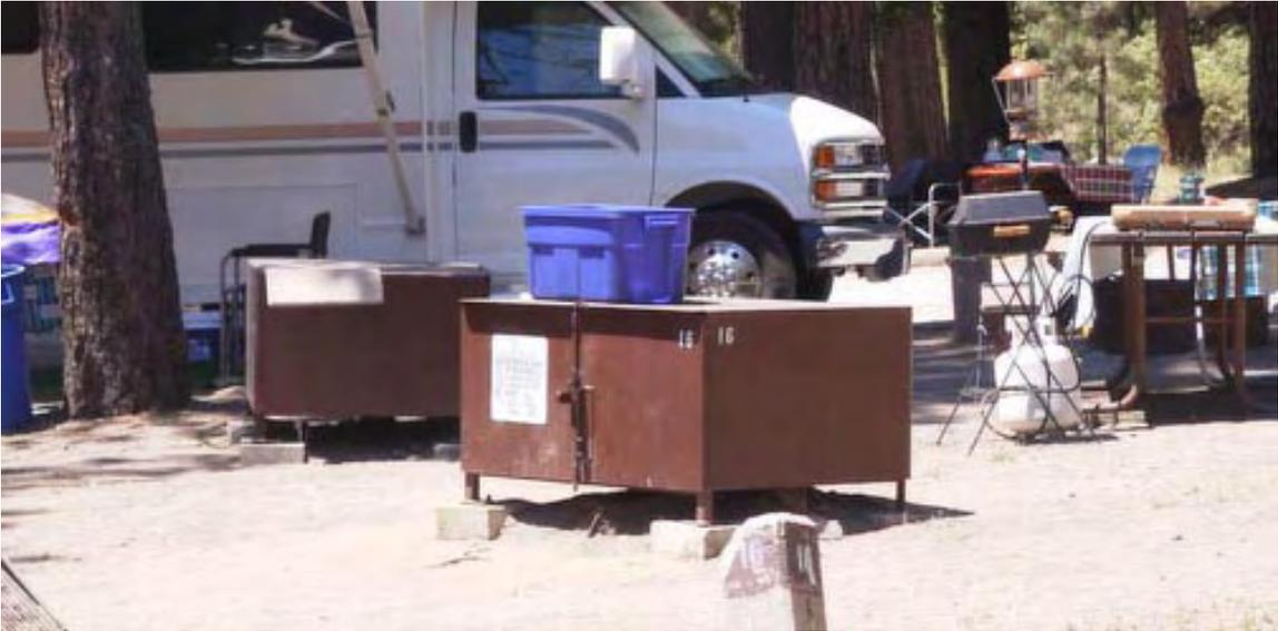
This is the “workhorse” bear box and by far the most common type of box in use in Yosemite National Park. The box itself measures 48 1/2” wide X 22 1/2” high and stands on legs that put the surface at 27” above ground level in most cases.
