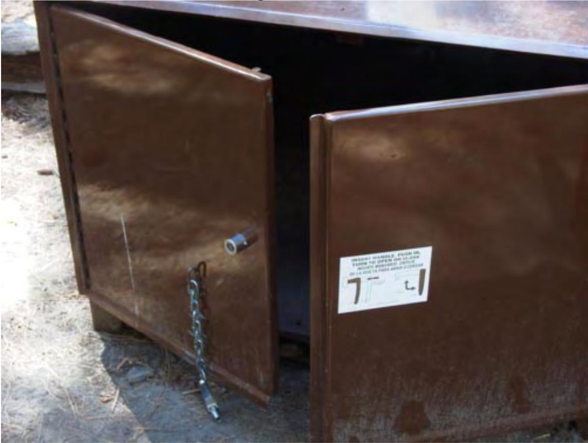
These “Bearnmaster” brand boxes are located at the Volunteer and Employee Campground at Yellow Pines. These are large double-door boxes with handles that are inserted over a rotating stud to latch. They are labeled with stickers explaining how the latch works.
