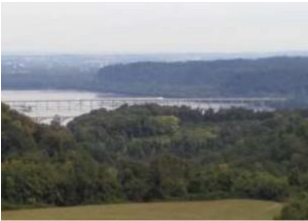
View of Susquehanna River, Columbia/Wrightsville Bridge and Route 30 Bridge.
