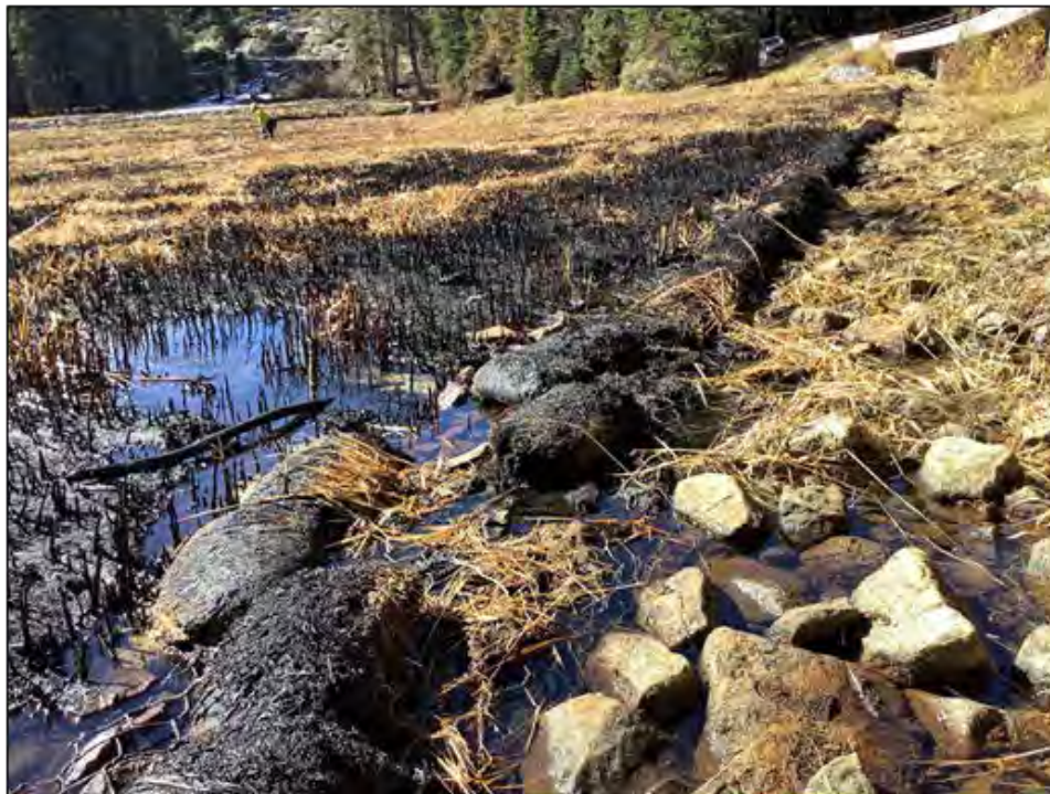
Figure 6. A row of sandbags designed to spread out surface flow in restored Halstead Meadow was damaged in the KNP Complex and started to fail in the October 25 storm.
