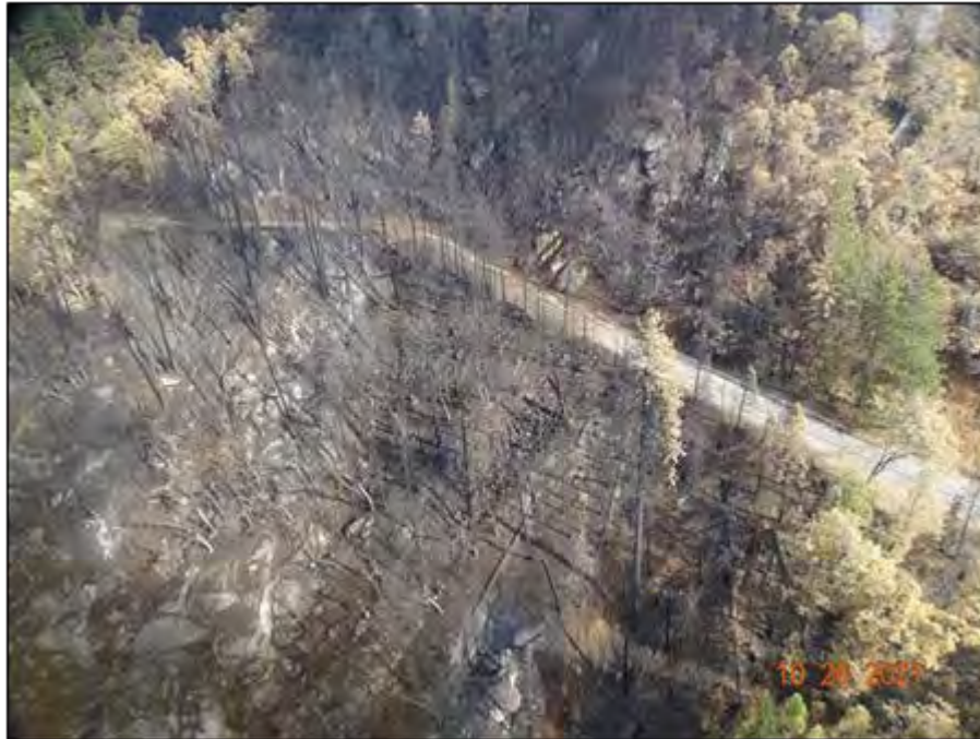
Photo 12 Generals Highway Historic District. View looking down from helicopter.
