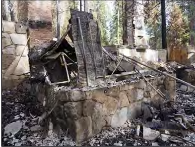
Photo 2 Redwood Mountain Ranger Station masonry remnants. View looking northeast.
