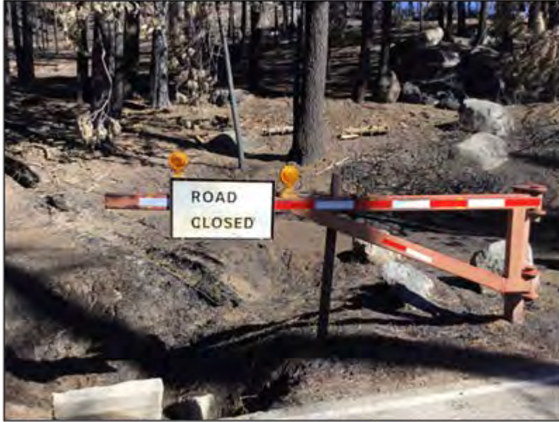
Permanent Road Closure Gate
