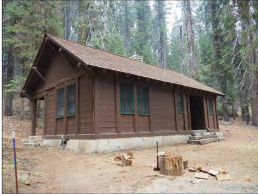
Photo 9 Cabin Creek Ranger Station. View looking northwest.
