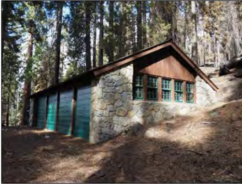
Photo 4 Redwood Mountain Garage/Equipment Shed. View looking west.
