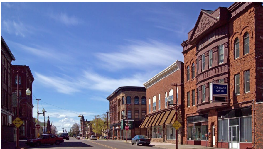
View south on Sixth Street, Calumet Civic Core. NPS photograph
