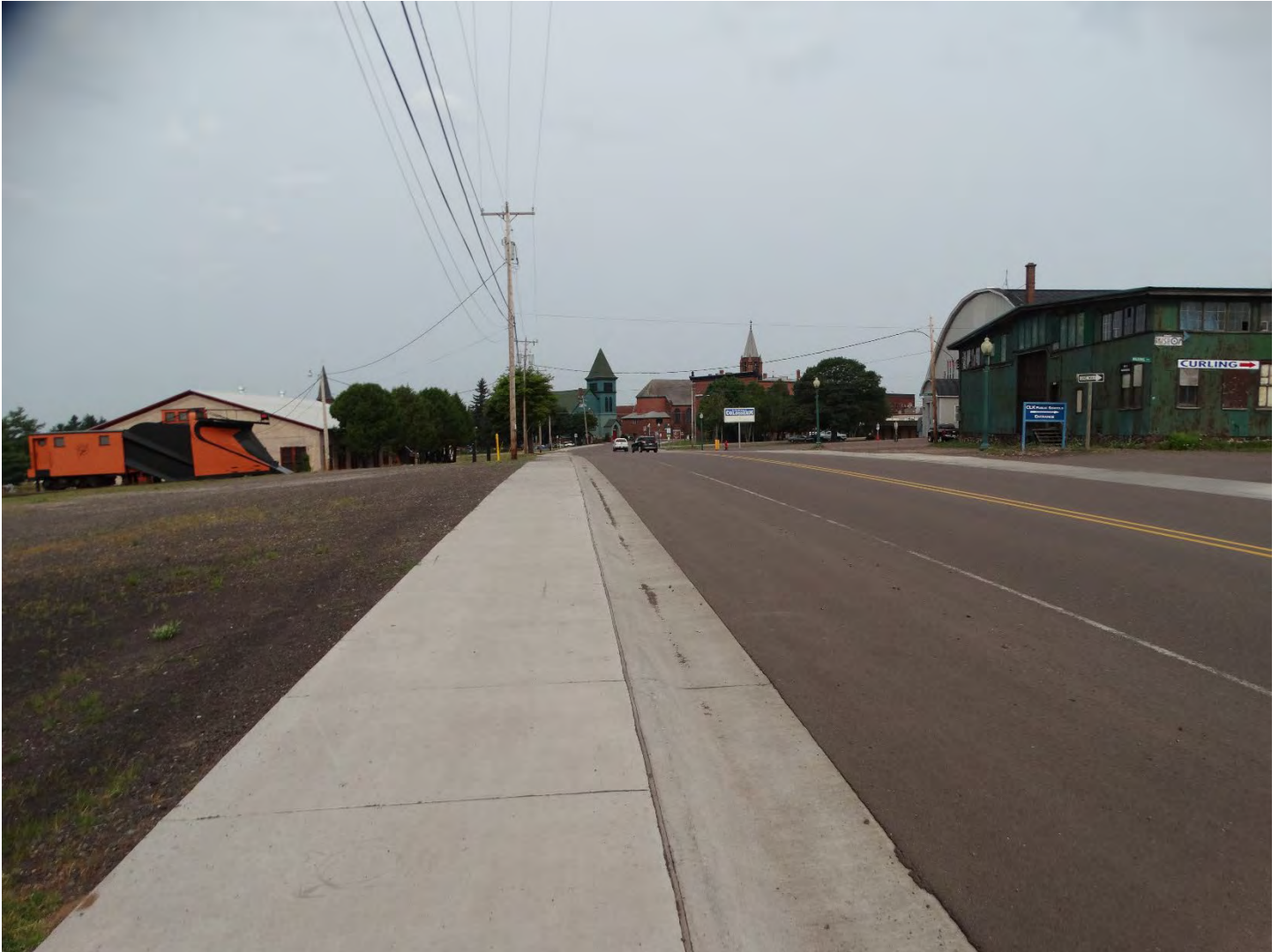
Calumet and Hecla Mine Industrial and Management Core Landscape Character Area A. The Russell Snow Plow (Map ID# 38) is on the left side of Red Jacket Road, the C& H Warehouse #2 (Map ID# 41) is on the right. Temple Square is in the distance.
