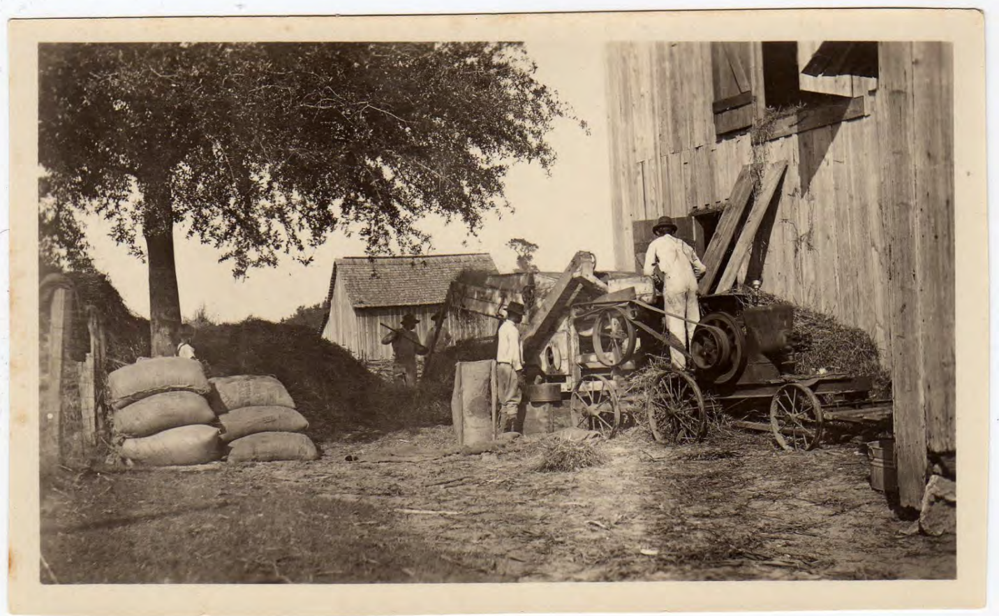
Figure 13. Threshing oats at east elevation of hay barn (#22), looking south with corn crib (#20) in background, c. 1915.
