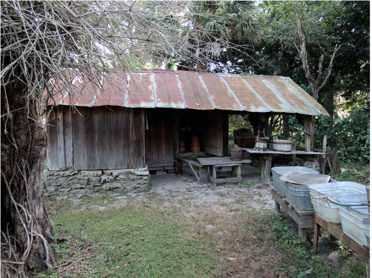
Photo 11 of 26 Dairy/canning shed (#11), looking east.
