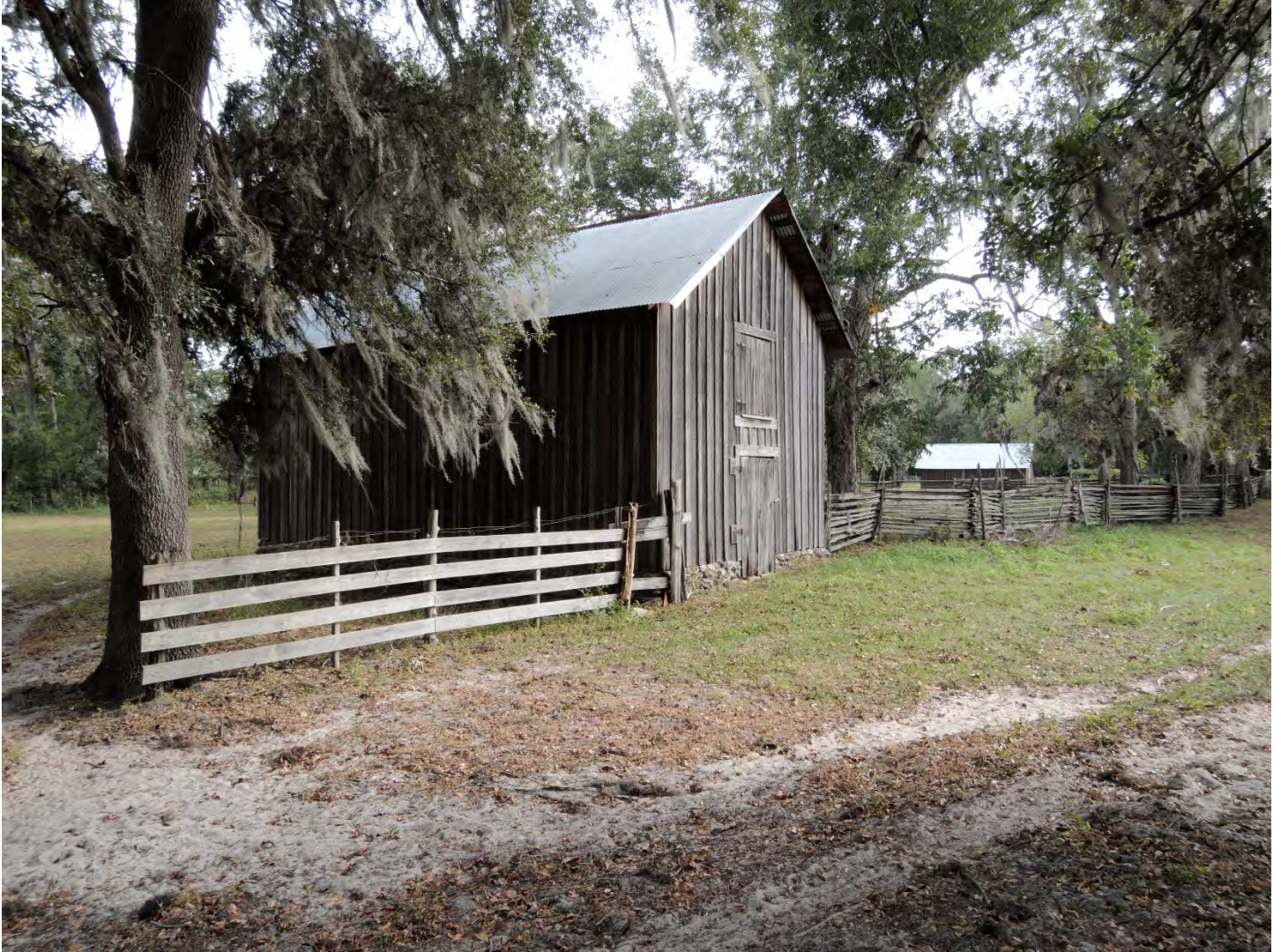
Photo 17 of 26 Hay barn (#22), looking southeast from road along western edge of farm complex.
