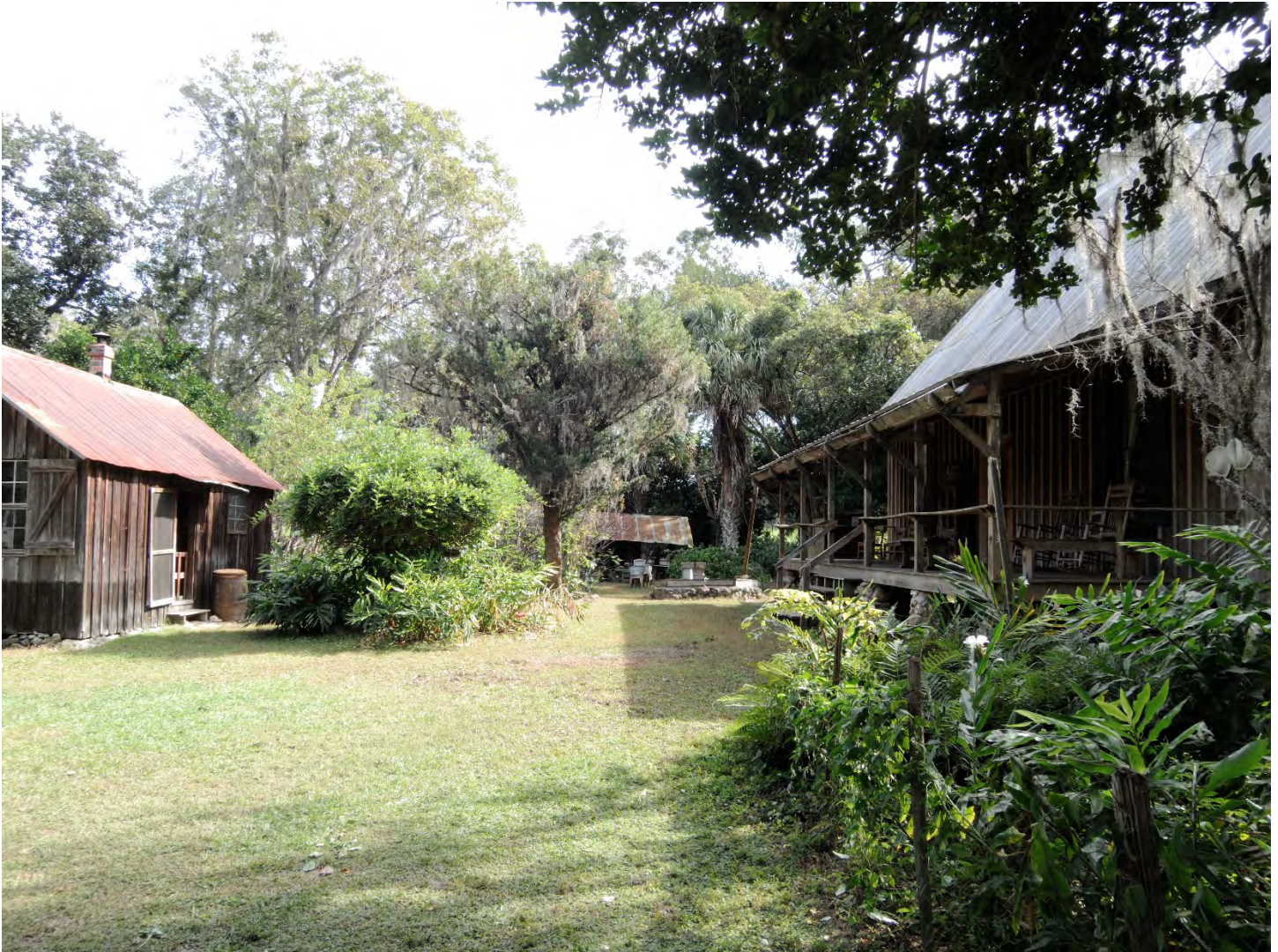
Photo 10 of 26 Rear yard of main house (#4), looking east, showing kitchen (#9) on left, dairy/canning shed (#11) in background, cistern (#8), and main house (#4) on right.
