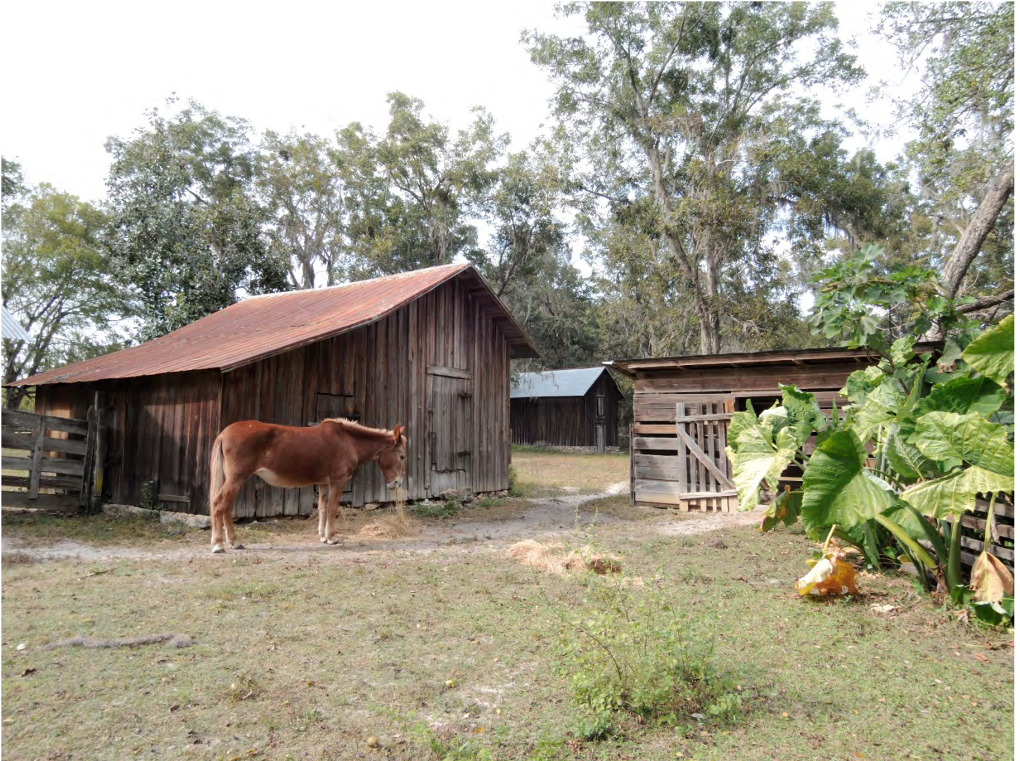
Photo 16 of 26 Mule lot, looking north showing corn crib (#20) on left, hay barn (#22) in background center, and mule stable (#21) on right.
