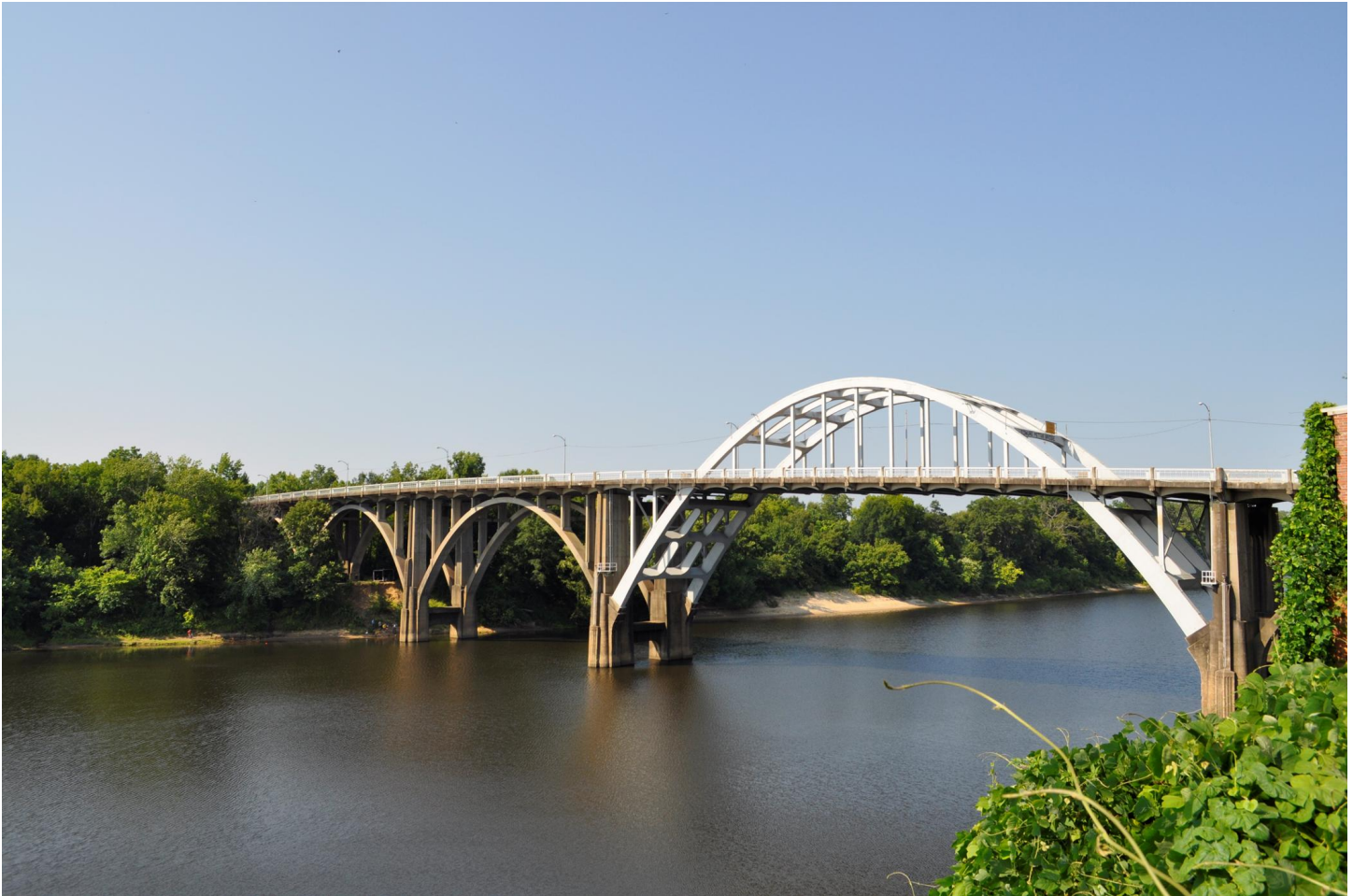
Edmund Pettus Bridge, camera looking northeast. Photograph by Cynthia Walton, Southeast Regional Office (SERO), National Park Service (NPS), June 26, 2012.
