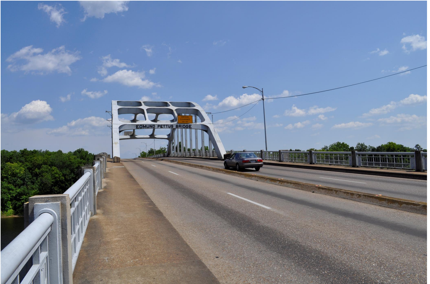
Edmund Pettus Bridge, camera looking south. Photograph by Cynthia Walton, SERO, NPS, June 26, 2012.
