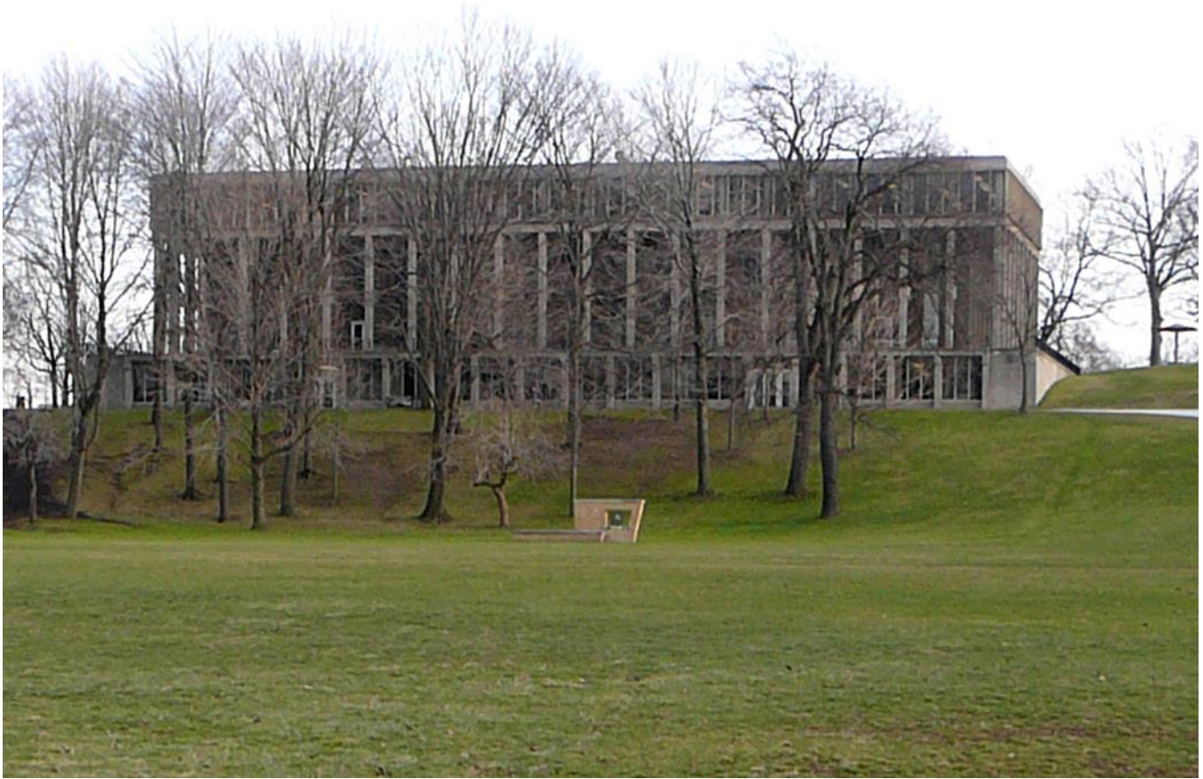
Photograph 6. Contributing building, Taylor Hall, facing southeast Photo by Mark Seeman, December 2006
