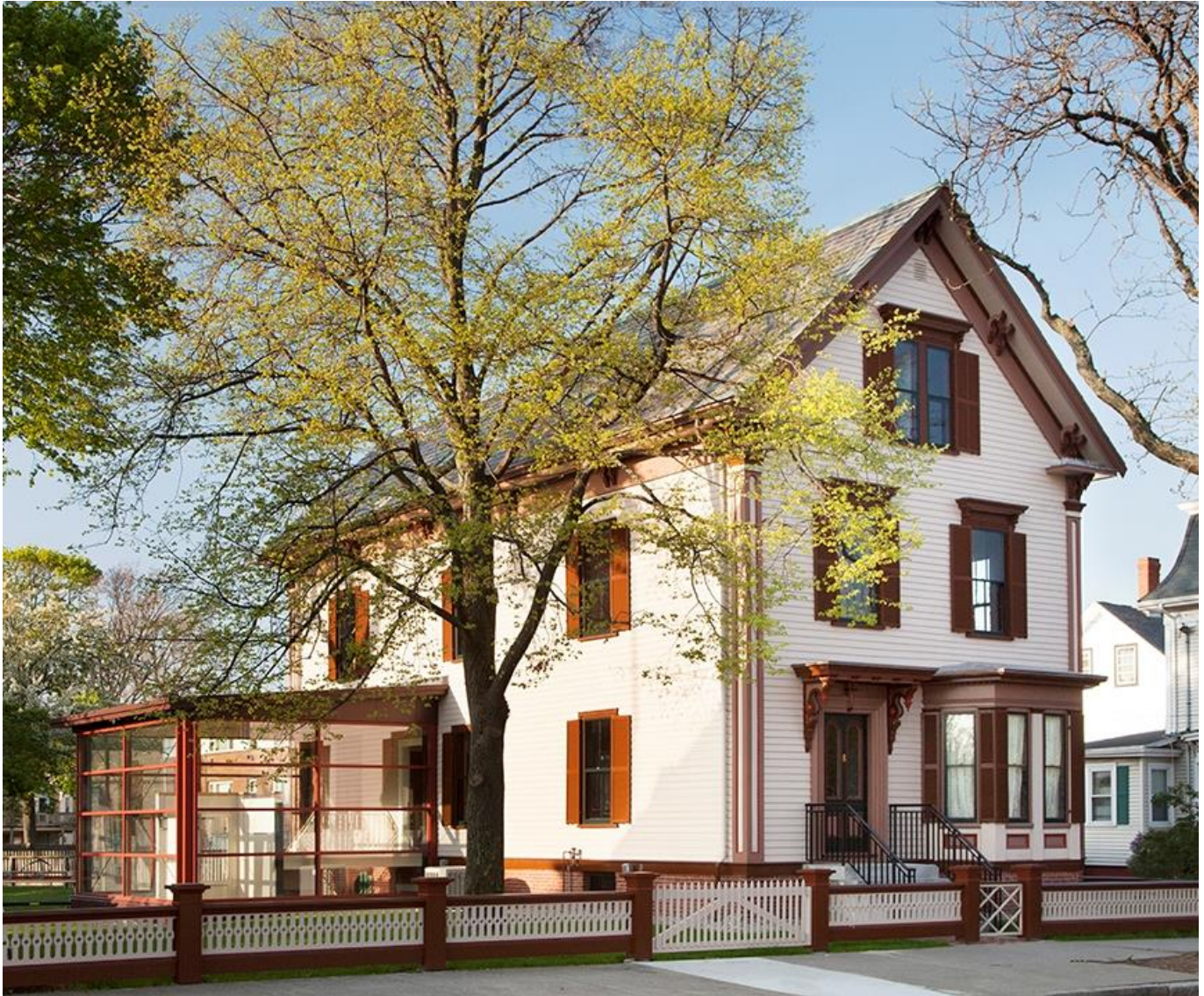
Image 8: Restored Mary Baker Eddy House with vestibule addition for universal accessibility, from northeast. Photo by Eric Roth, 2012.
