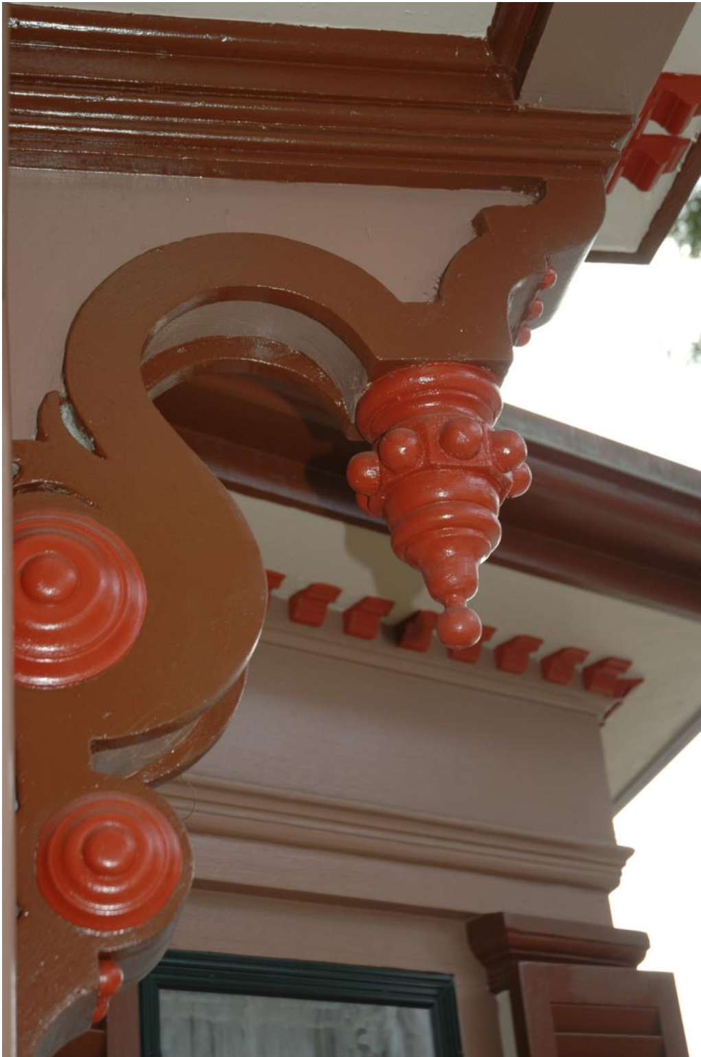
Image 13: Detail of restored drop bracket with historic colors.
