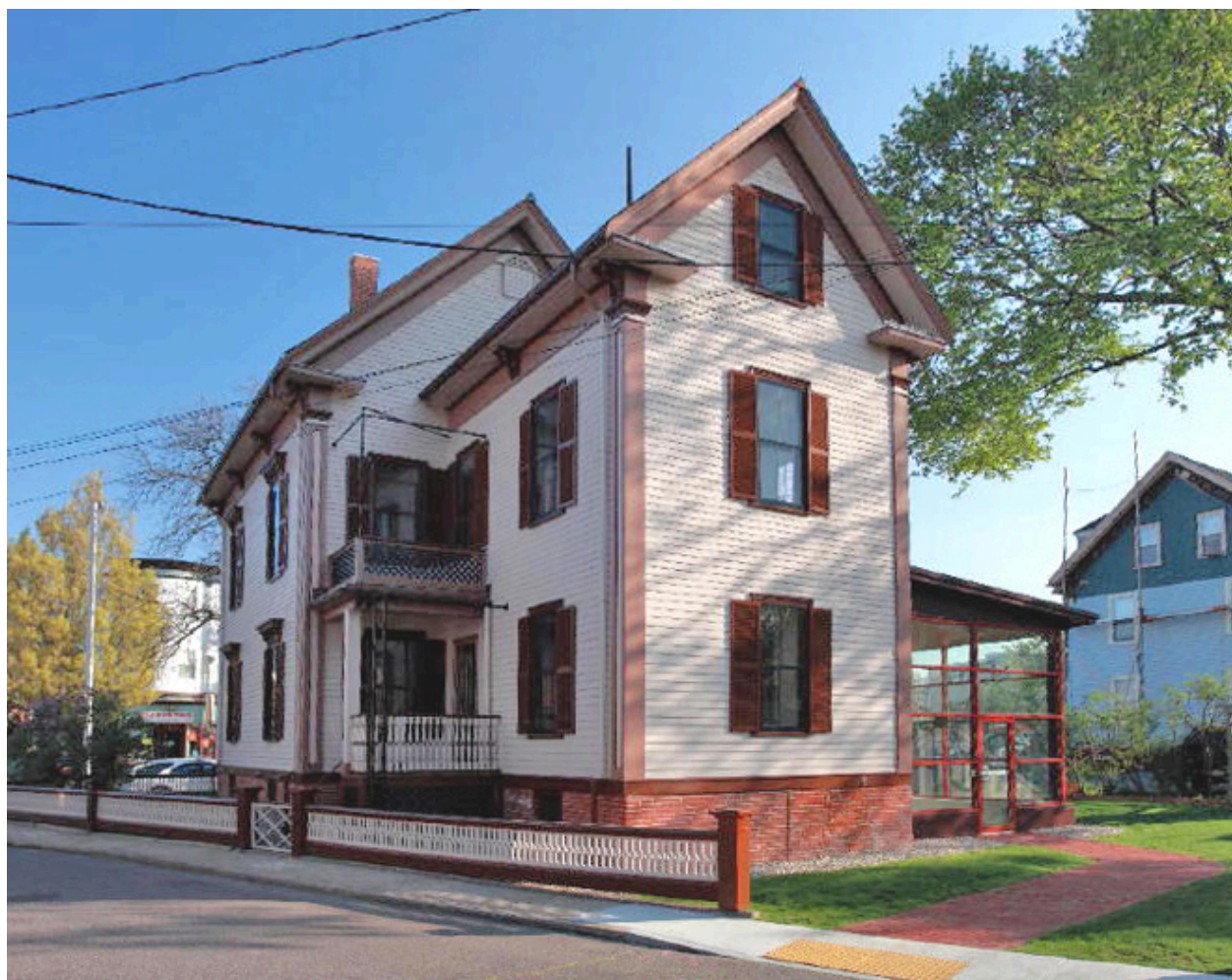
Image 11: Restored Mary Baker Eddy House, from southwest. Photo by Eric Roth, 2012.
