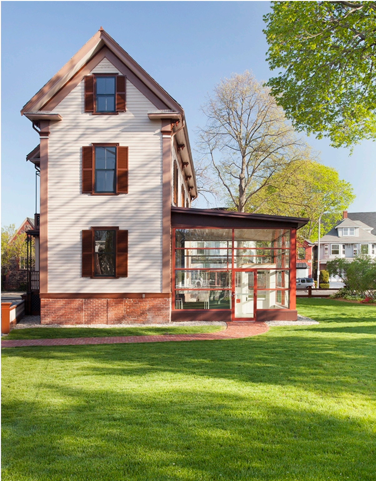
Image 10: Restored Mary Baker Eddy House with vestibule addition for universal accessibility, south façade. Photo by Eric Roth, 2012.
