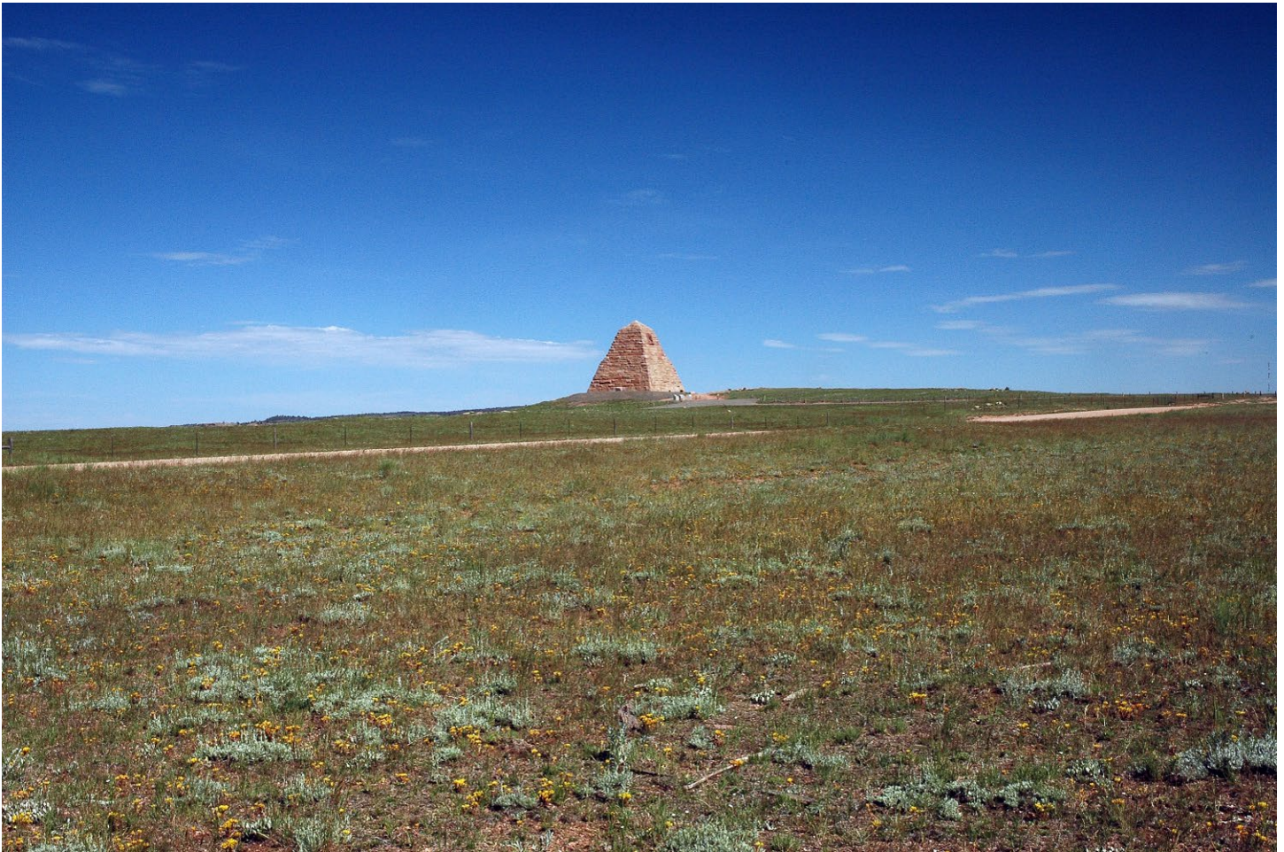
Photo 6. Ames Monument, south and east elevations. Richard Collier, photographer, June 2014
