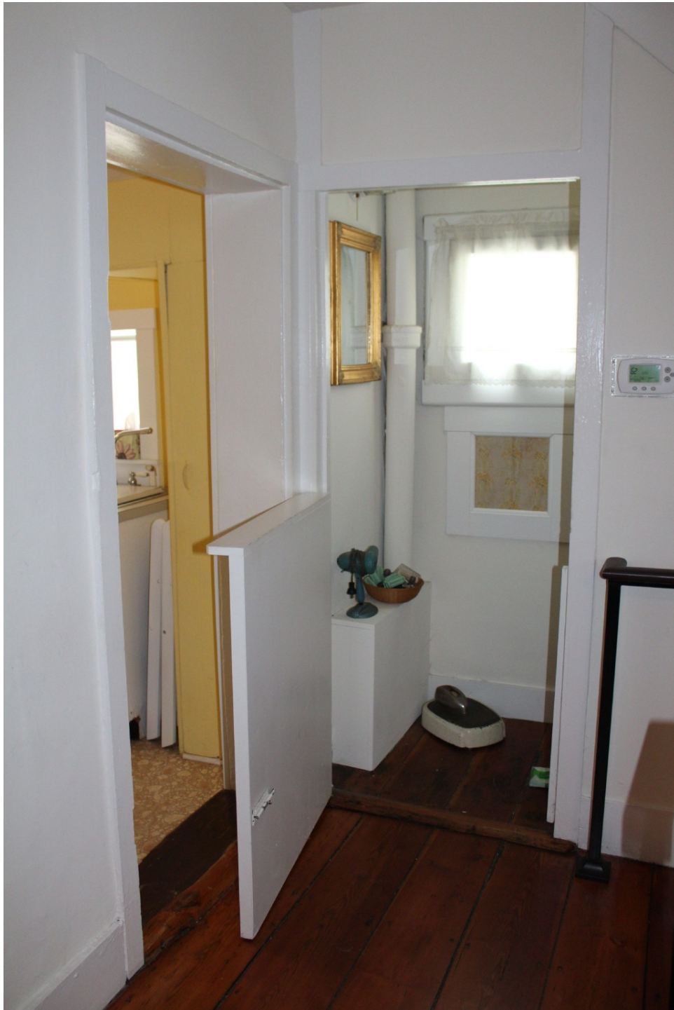
Photo 9. Bathroom on first floor, looking southeast; door to kitchen is on left. April 2018.
