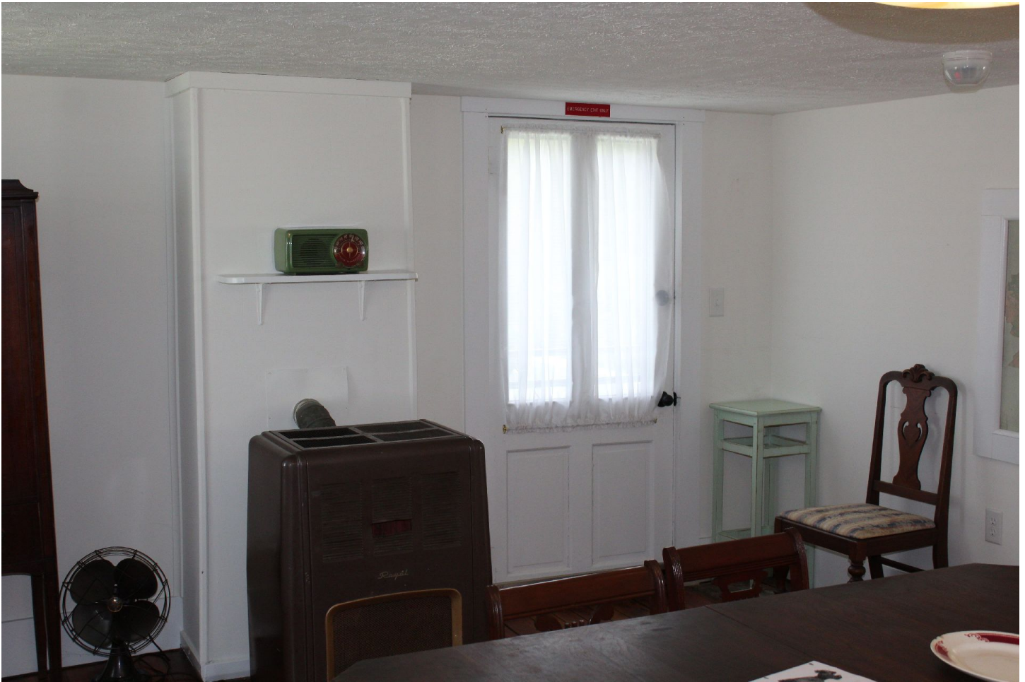
Photo 13. Dining room on first floor, looking southeast, showing back door and chimney stack. April 2018.
