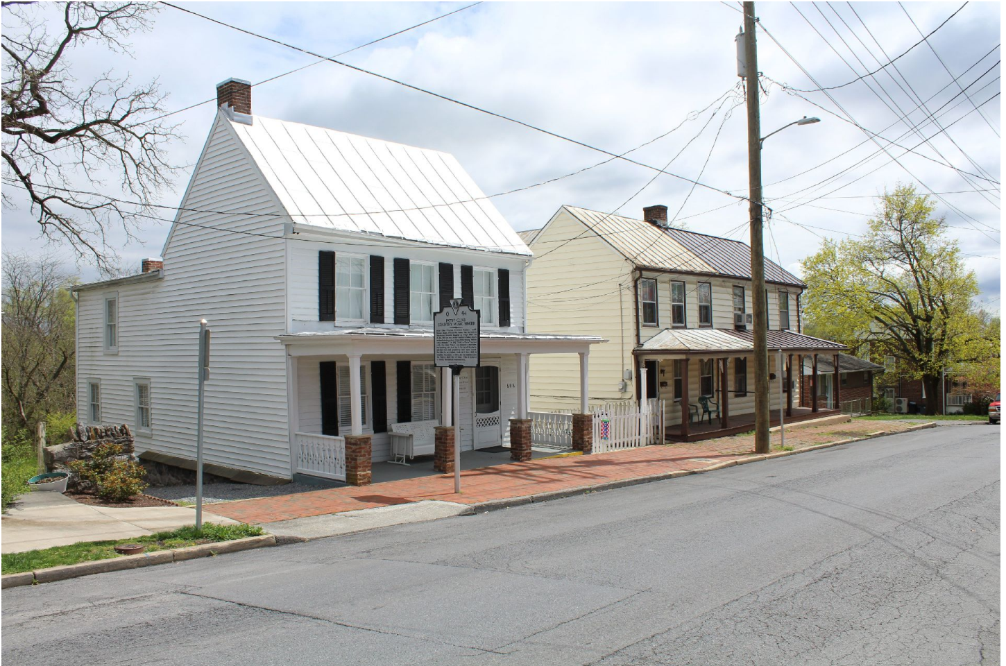
Photo 1. Exterior, looking southeast from South Kent Street, showing setting and north and west elevations. April 2018.
