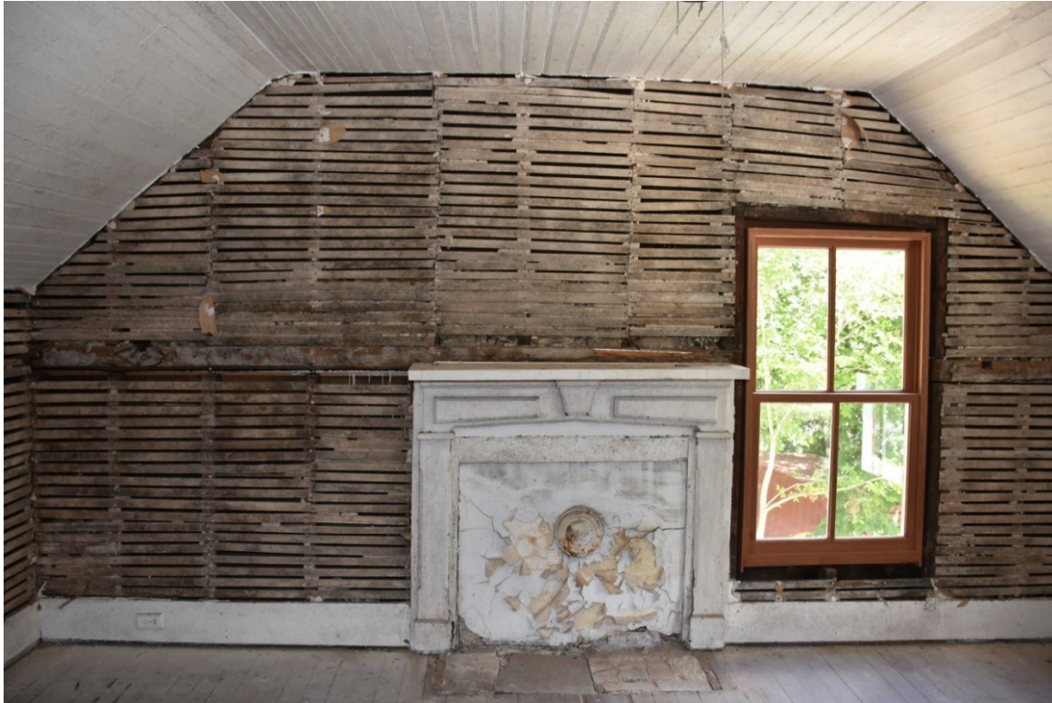
8. Second floor, north bedroom, looking north (above)
