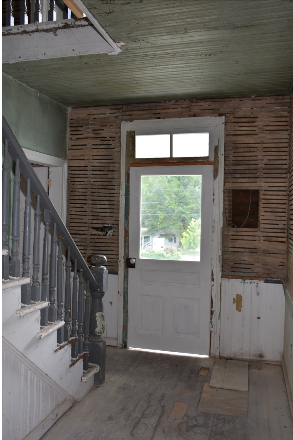
5. First floor, center hall, looking east
