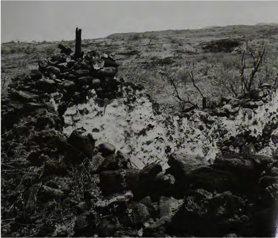
Figure 32. John Young's main house around 1964. The original wood support beams remain embedded in a collapsed wall. Photograph courtesy of NPS.
