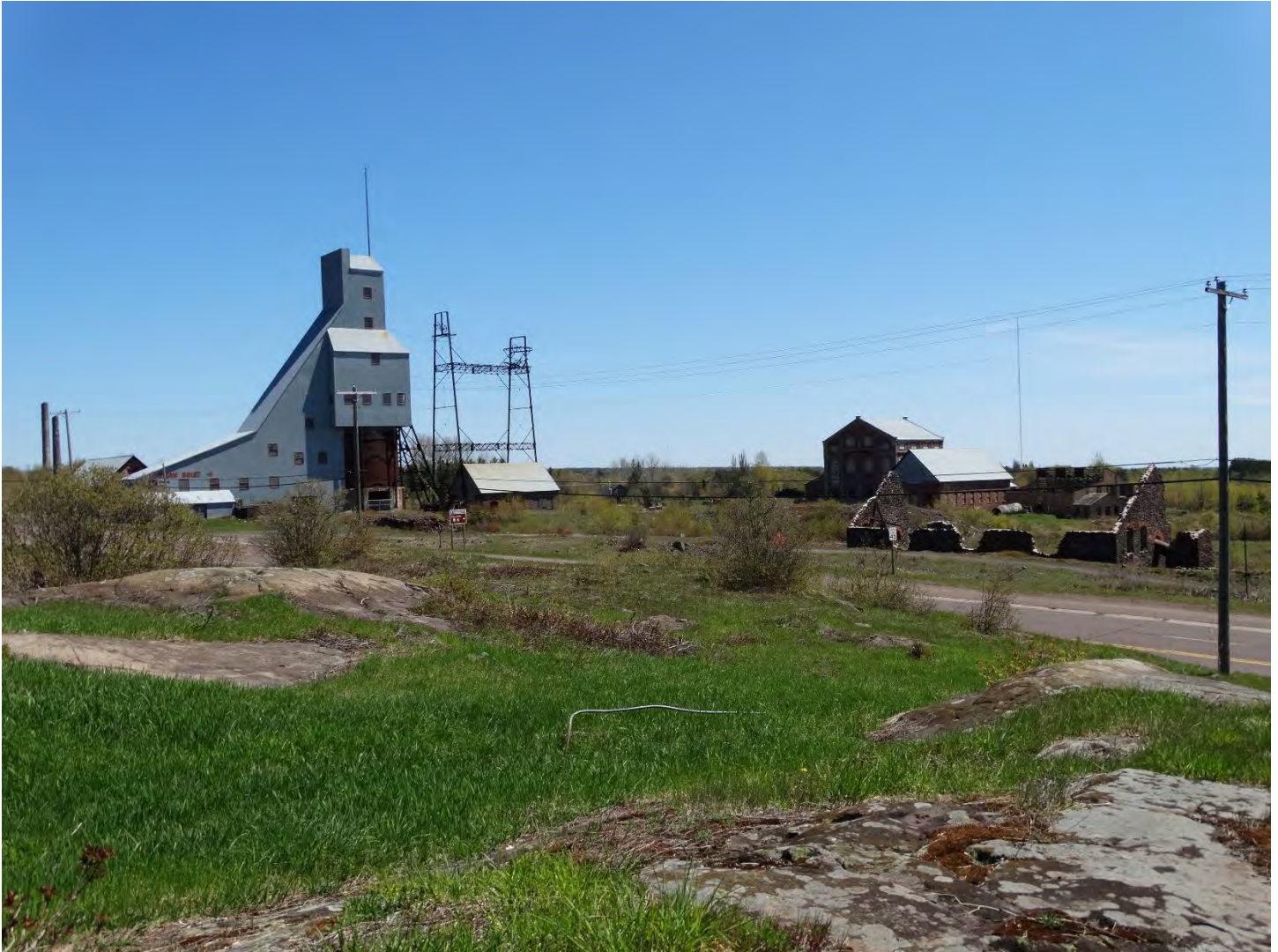
Quincy Mine Industrial Core Landscape Character Area 1. Left to right: the No. 2 Shaft-Rockhouse (Map ID# 006), Pulley Stand (MAP ID# 007), 1882 No. 2 Hoist House (MAP ID# 008), the 1918-1920 No. 2 Hoist House (MAP ID# 012), and the 1894-1985 No. 2 Hoist House (MAP ID# 013). The No. 4 Boiler House Ruin (MAP ID# 005) is in the right, middle ground.
