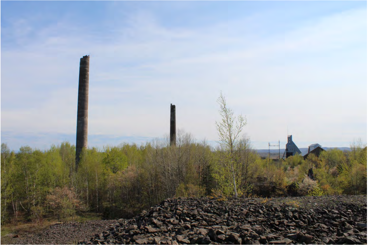
Quincy Mine Industrial Core Landscape Character Area 1. Poor rock pile in the No. 6 area; the No. 6 Boiler House Stack (MAP ID#26), and the No. 2 Boiler House Stack (Map ID# 025) on the left. The roof of the Quincy Machine Shop (MAP ID# 023) and the No. 2 Shaft-Rockhouse (Map ID# 006) are in the distance.
