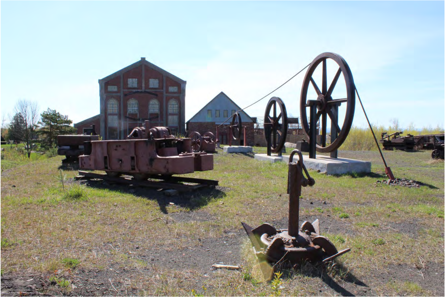
Quincy Mine Industrial Core Landscape Character Area 1. Left to right: the 1918-1920 No. 2 Hoist House (MAP ID# 012), the 1894-1985 No. 2 Hoist House (MAP ID# 013) and three pulleys (MAP ID# 011).
