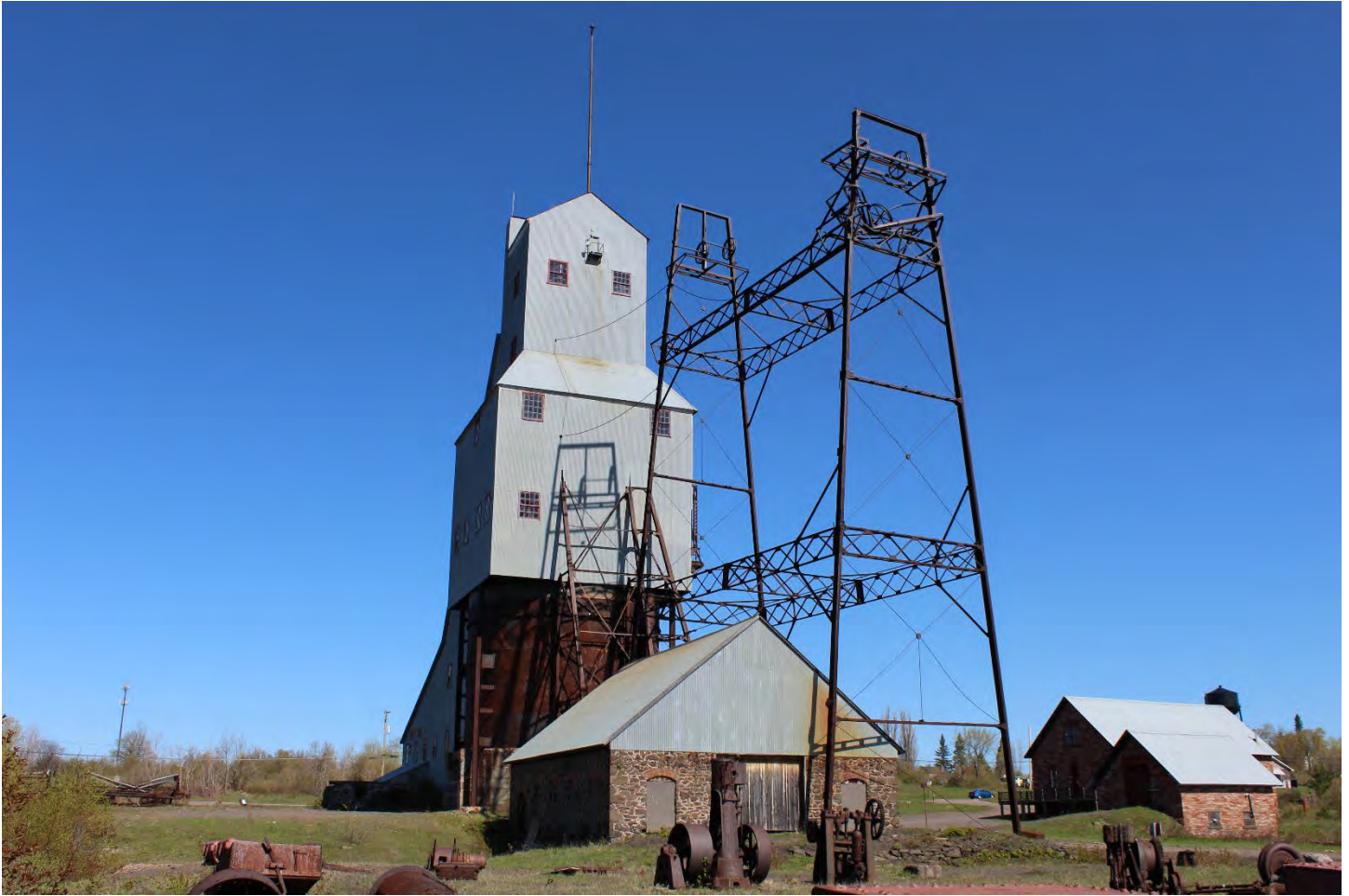
Quincy Mine Industrial Core Landscape Character Area 1. The No. 2 Shaft-Rockhouse (Map ID#006) is in the center background, the 1882 No. 2 Hoist House (Map ID# 008) and Pulley Stand (MAP ID# 007) in the center, the Oil House (MAP ID# 010) and Supply Office (MAP ID# 009) to the right.
