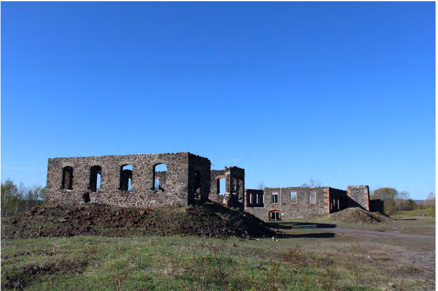
Quincy Mine Industrial Core Landscape Character Area 1. Left to right: No. 4 Boiler House Ruin (Map ID# 004) and the No. 7 Boiler House Ruin (Map ID#003).
