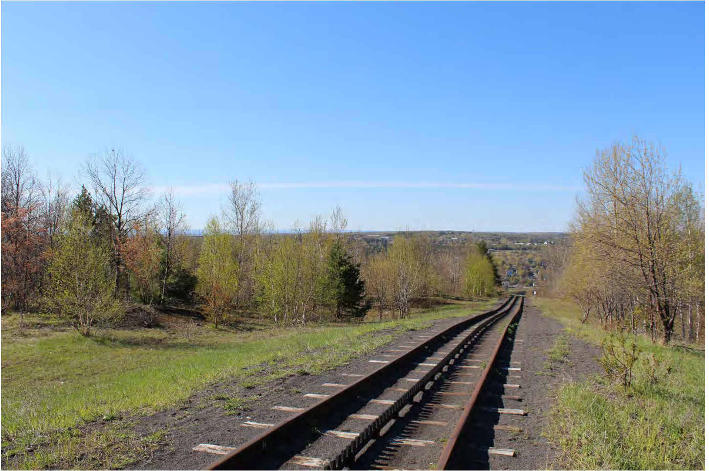
Quincy Mine Industrial Core Landscape Character Area 1. Tram at No. 2 area looking south toward Hancock.
