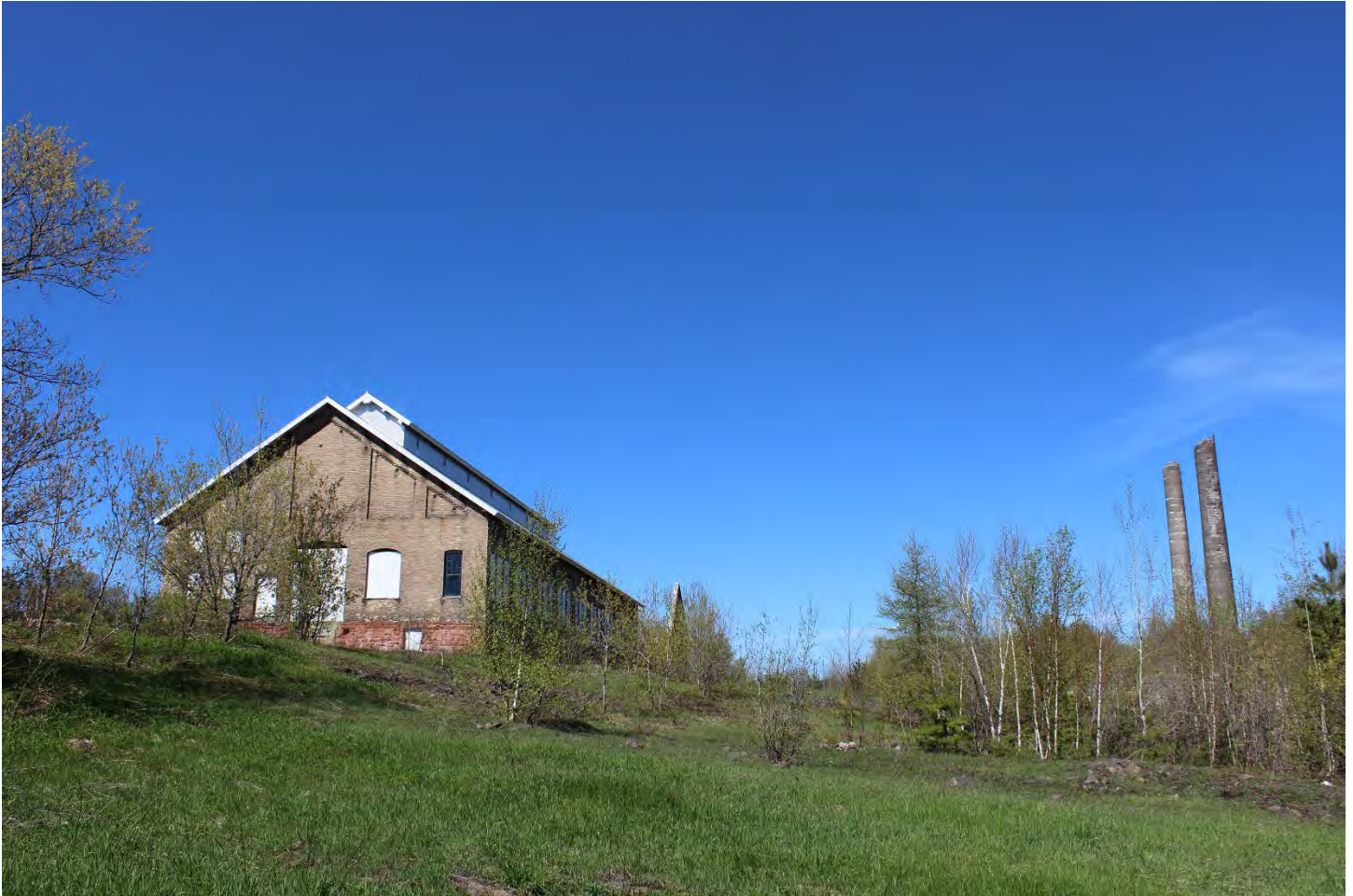
Quincy Mine Industrial Core Landscape Character Area 1. South end and east side of the Quincy Machine Shop (MAP ID# 023), the No. 2 Boiler House Stack (Map ID# 025) and the No. 6 Boiler House Stack (MAP ID#26) in the distance.
