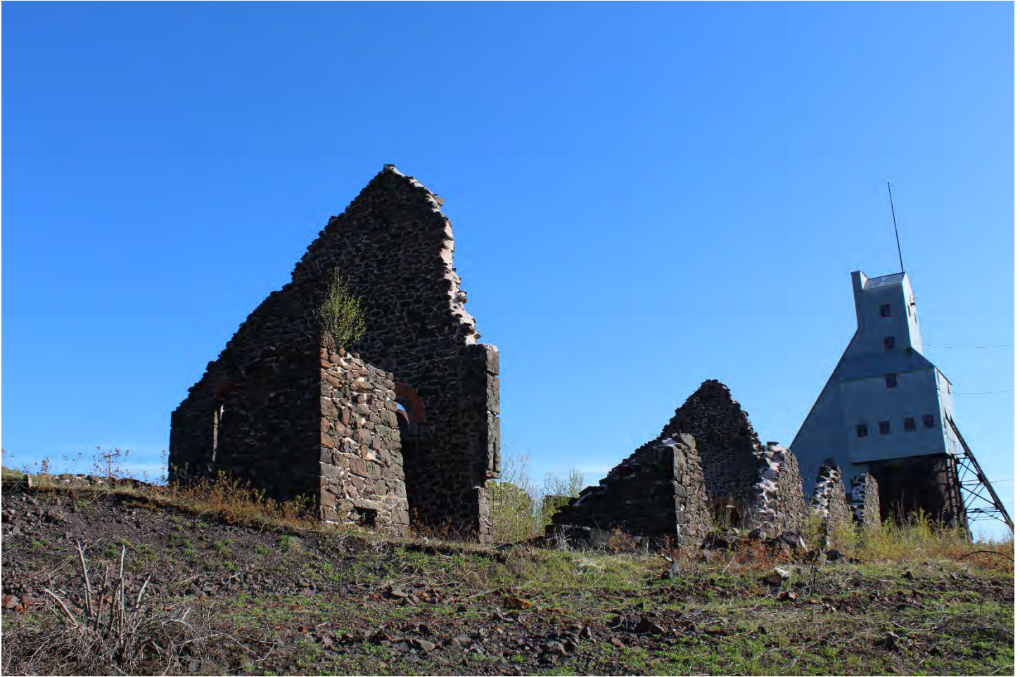
Quincy Mine Industrial Core Landscape Character Area 1. Left to right: No. 5 Boiler House Ruin (Map ID# 005) and the No. 2 Shaft-Rockhouse (Map ID# 006).
