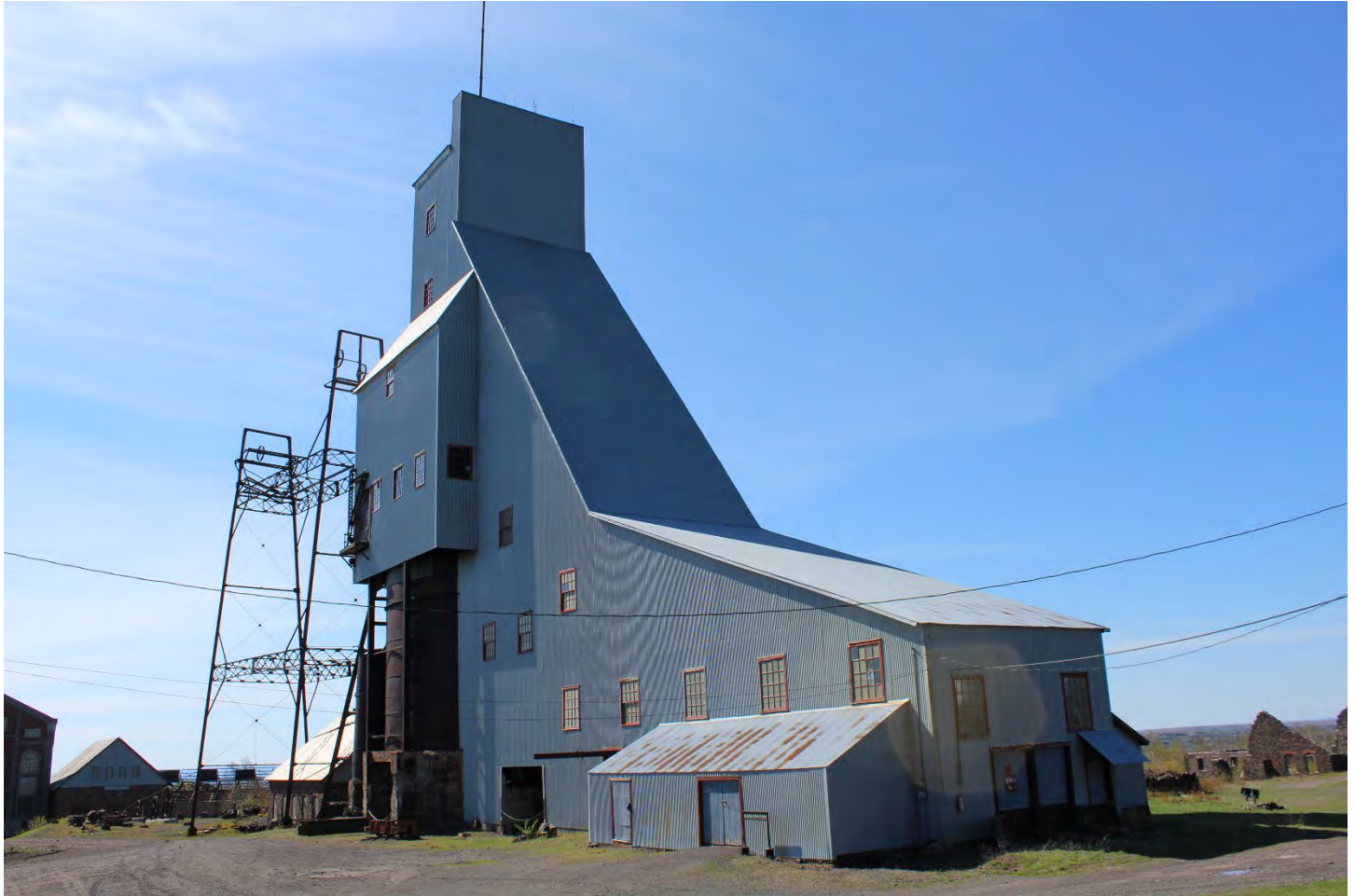
Quincy Mine Industrial Core Landscape Character Area 1. The No. 2 Shaft-Rockhouse (Map ID# 006), Pulley Stand (MAP ID# 007) to the rear.
