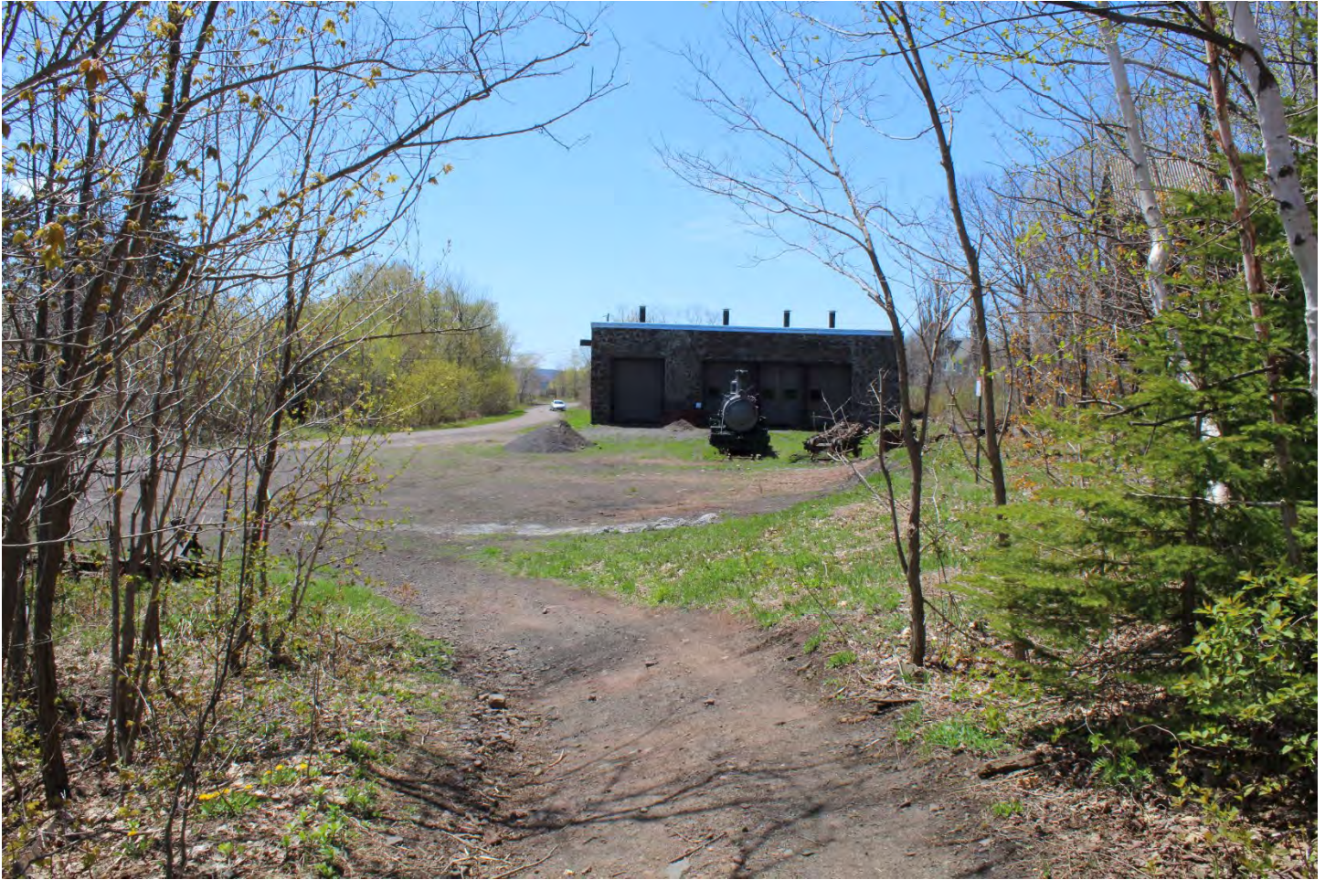
Quincy Mine Industrial Core Landscape Character Area 1. The Quincy and Torch Lake Railroad Engine House (MAP ID# 001) and remnants of rolling stock.
