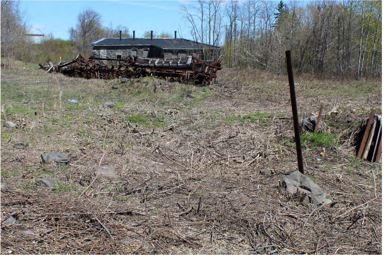
Quincy Mine Industrial Core Landscape Character Area 1. The Quincy and Torch Lake Railroad Engine House (MAP ID# 001) and remnants of rolling stock.
