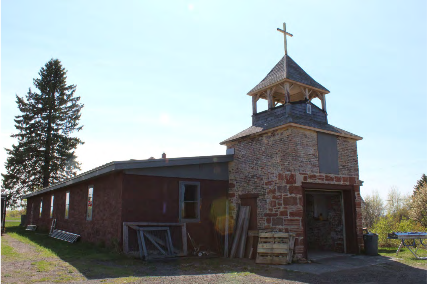
Quincy Hill Housing and Mine Management Landscape Character Area 2. Limerick Housing Location, former Catholic Church on E. 2 nd Street (MAP ID# 095).
