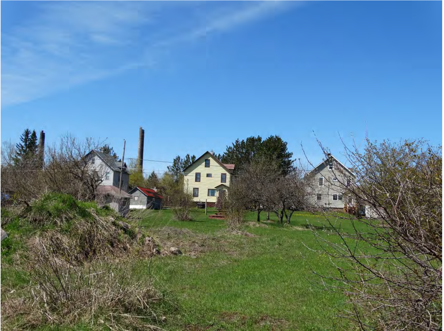
Lower Pewabic Housing Location Landscape Character Area 3. Back of residences along West Lower Pewabic Street (left to right: MAP ID#s 132, 133 and 134). The No. 6 and No. 2 Boiler House Stacks (MAP ID# 026 and 025) in the distance, left.
