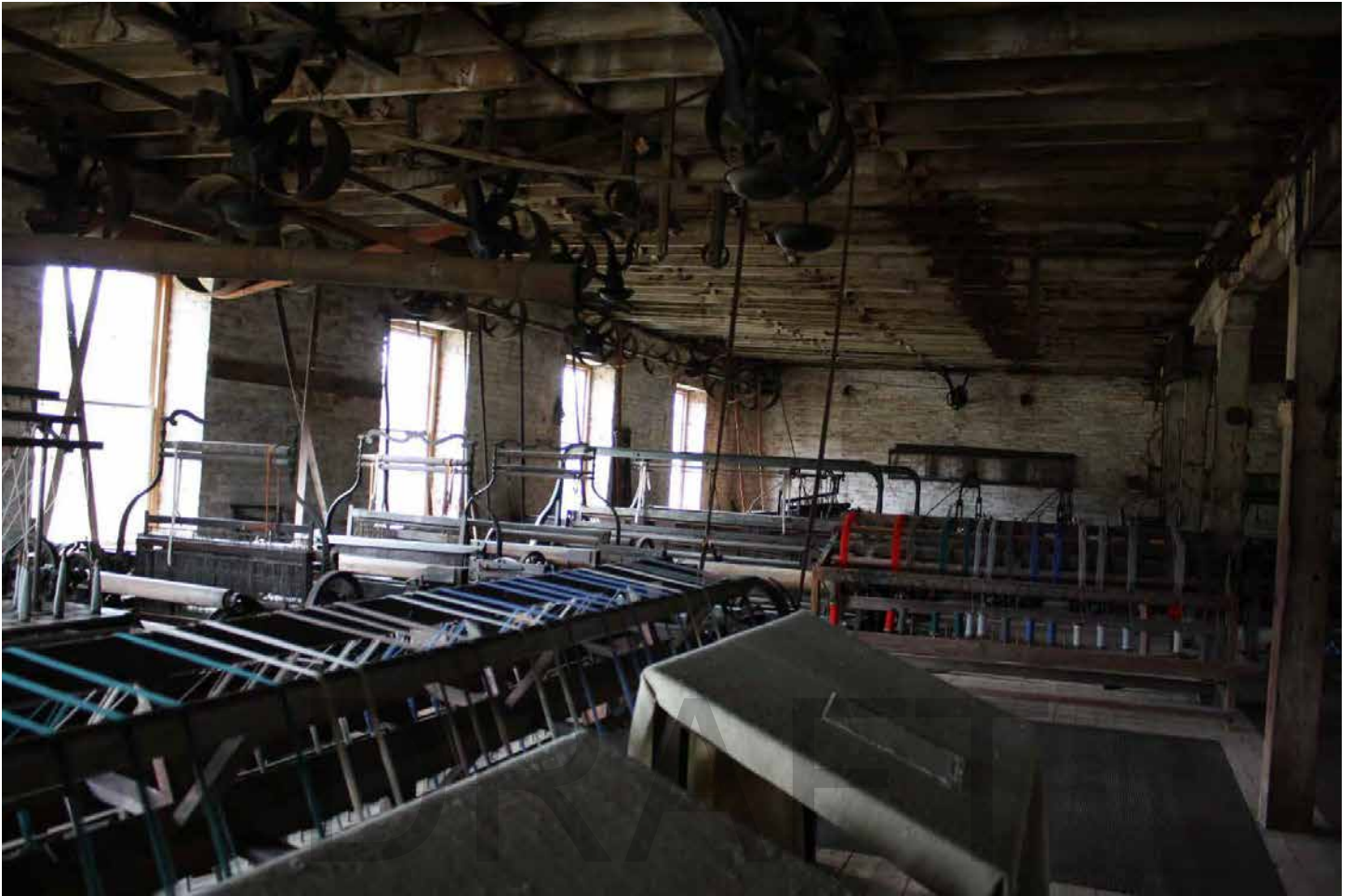
Photo 0020 MO_Clay County_Watkins Mill_0020 Watkins Mill, second floor, weaving room, camera facing east
