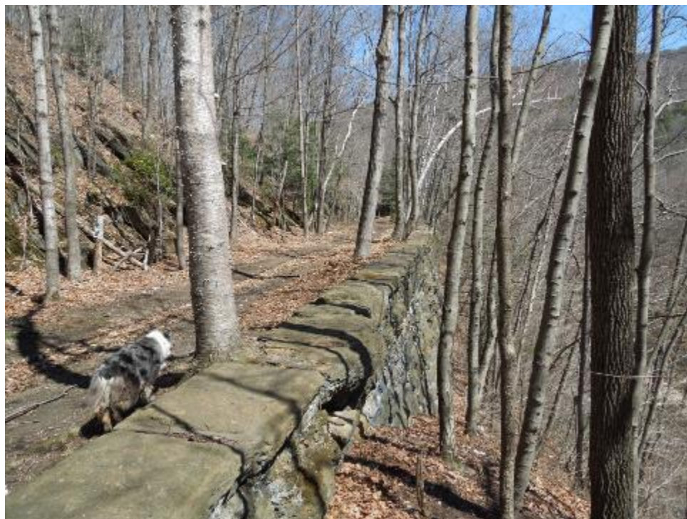
9. Embankment and retaining wall of Western Railroad Roadbed between Bridges No. 5 and 6, looking east. Roger Reed, NPS, 2014.
