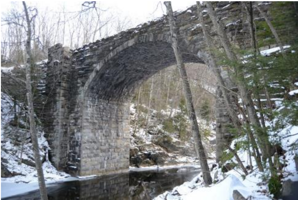
12. North side of Bridge No. 5, looking southeast. John Daly, PAL, 2017.
