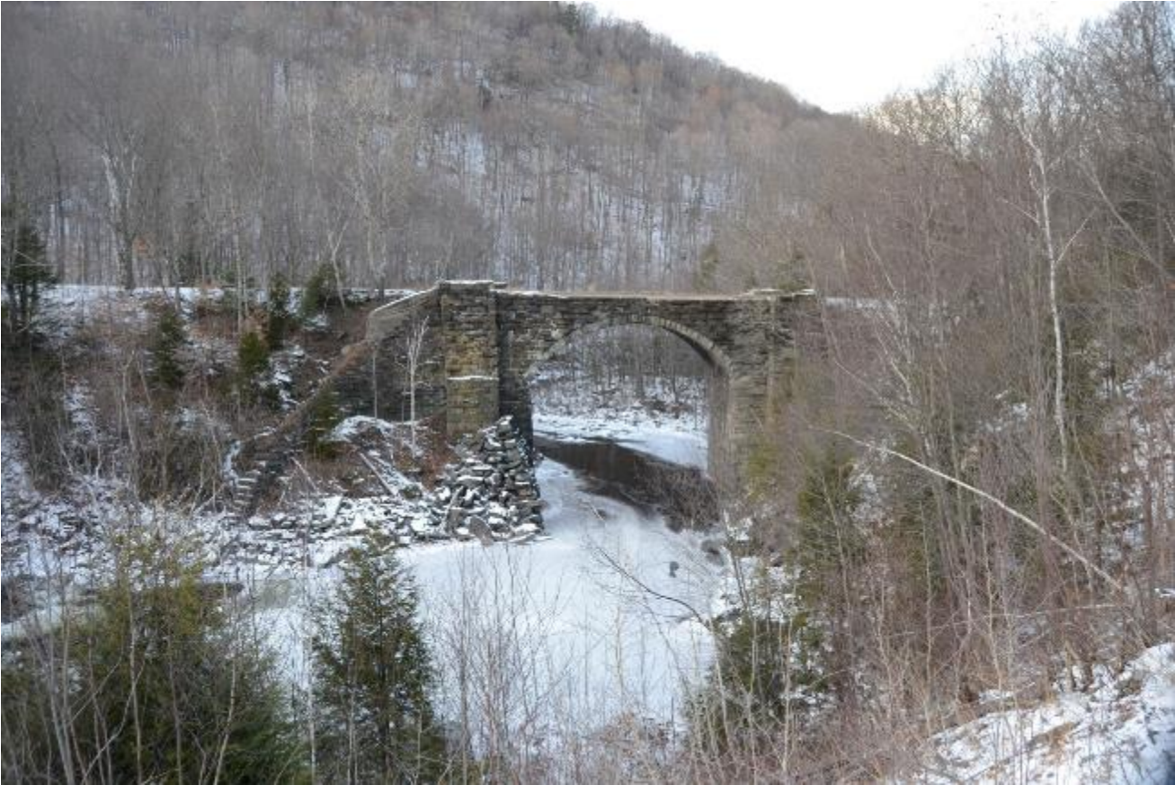
10. Western Railroad Roadbed and Western Railroad Stone Arch Bridge No. 5 (Bridge No. 5) in the Westfield River gorge, looking north (downstream). John Daly, PAL 2017.
