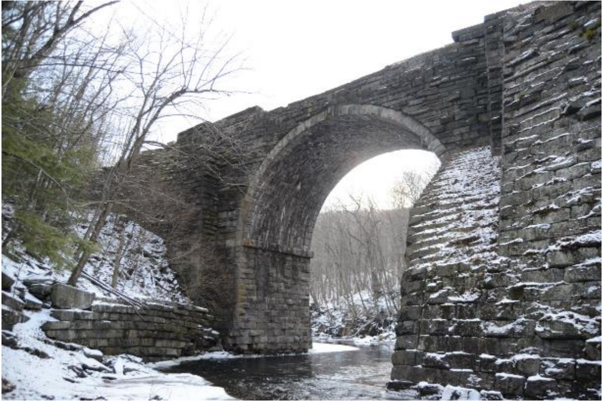
5. Northeast elevation of Bridge No. 6, looking south. John Daly, PAL, 2017.
