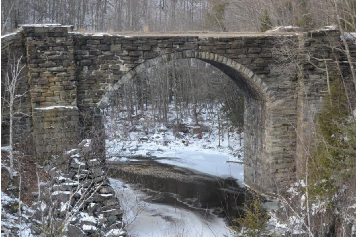
11. South side of Bridge No. 5, looking north. John Daly, PAL, 2017.
