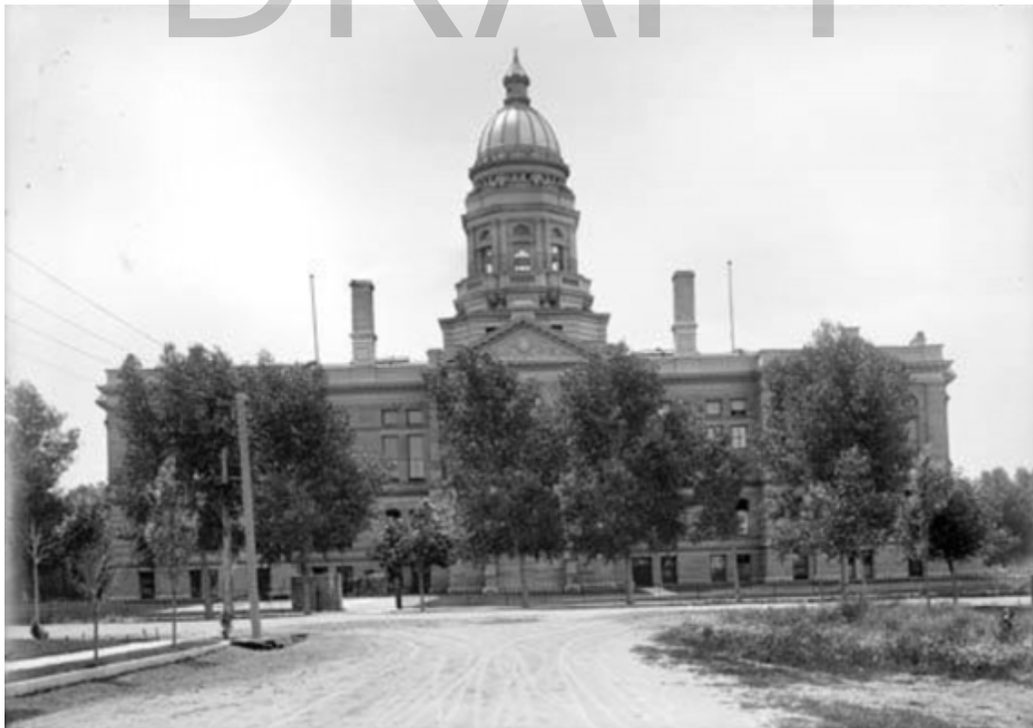
Figure 19: Capitol, north side between 1906 and 1917. Structure near the street edge in the service area west of the entrance was likely an ash pit. Photographer unknown. (Wyoming State Archives/WATS/15)
