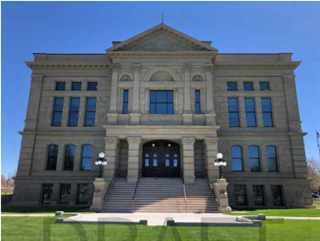
Photo 8 of 55: West side. Camera facing east. May 2021.
