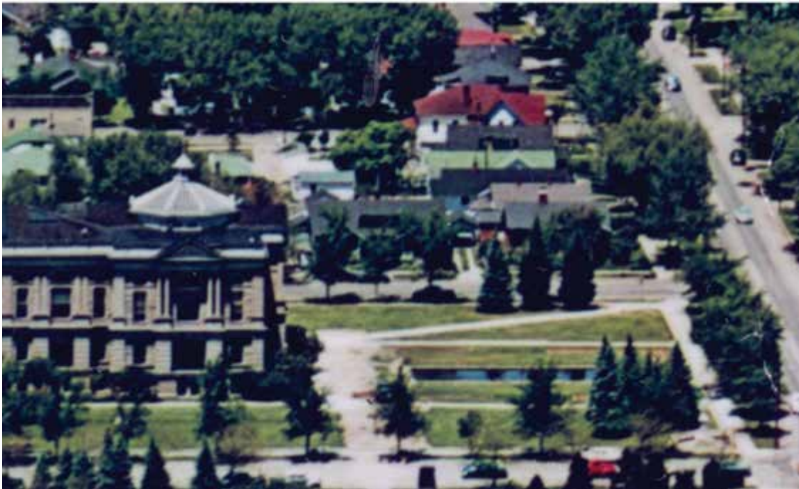
Figure 32: Aerial photograph of the Capitol grounds, east lawn, ca. 1940. Note the rectilinear reflecting pool. (Original source unknown/Wyoming State Capitol Renovation & Restoration Level I Reconnaissance & Level II Feasibility Study, 2013-2014)
