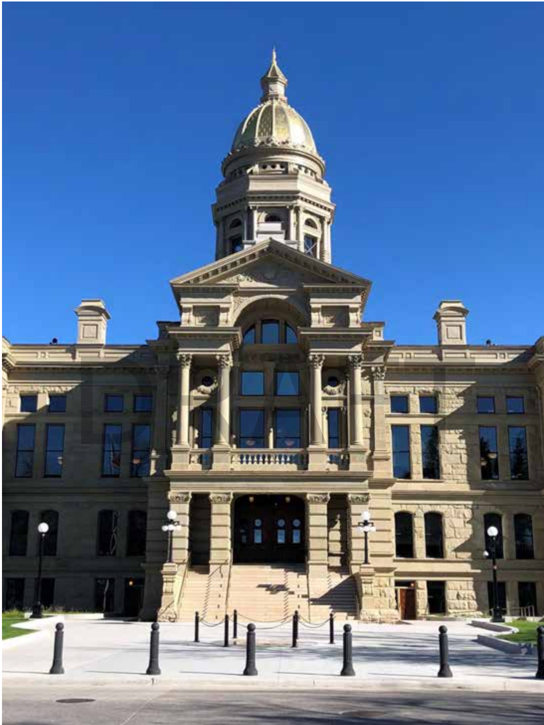
Photo 5 of 55: South side, monumental main entrance pavilion. Camera facing north. May 2021.
