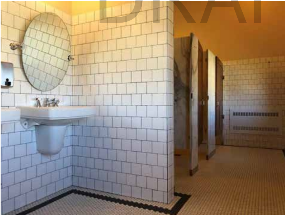
Photo 42 of 55: Non-historic restrooms have been compatibly designed to maintain the Capitol's historic feeling. The marble used to construct the stall dividers was quarried from the same source used to procure the marble for the historic flooring throughout the building.
