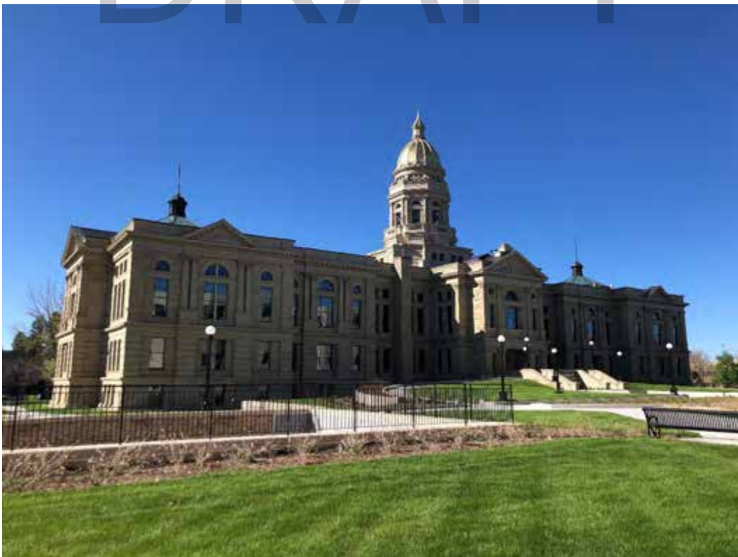
Photo 9 of 55: North side. Camera facing southwest. May 2021.
