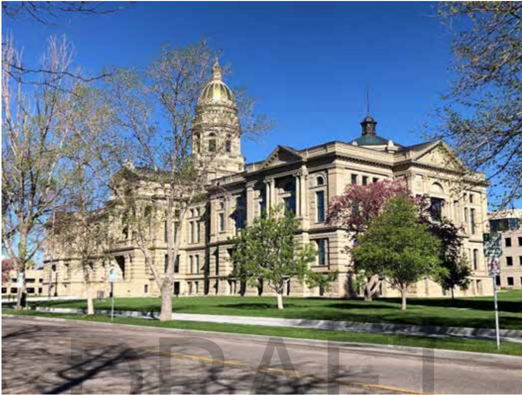
Photo 15 of 55: South and east sides. Camera facing northwest. May 2021.
