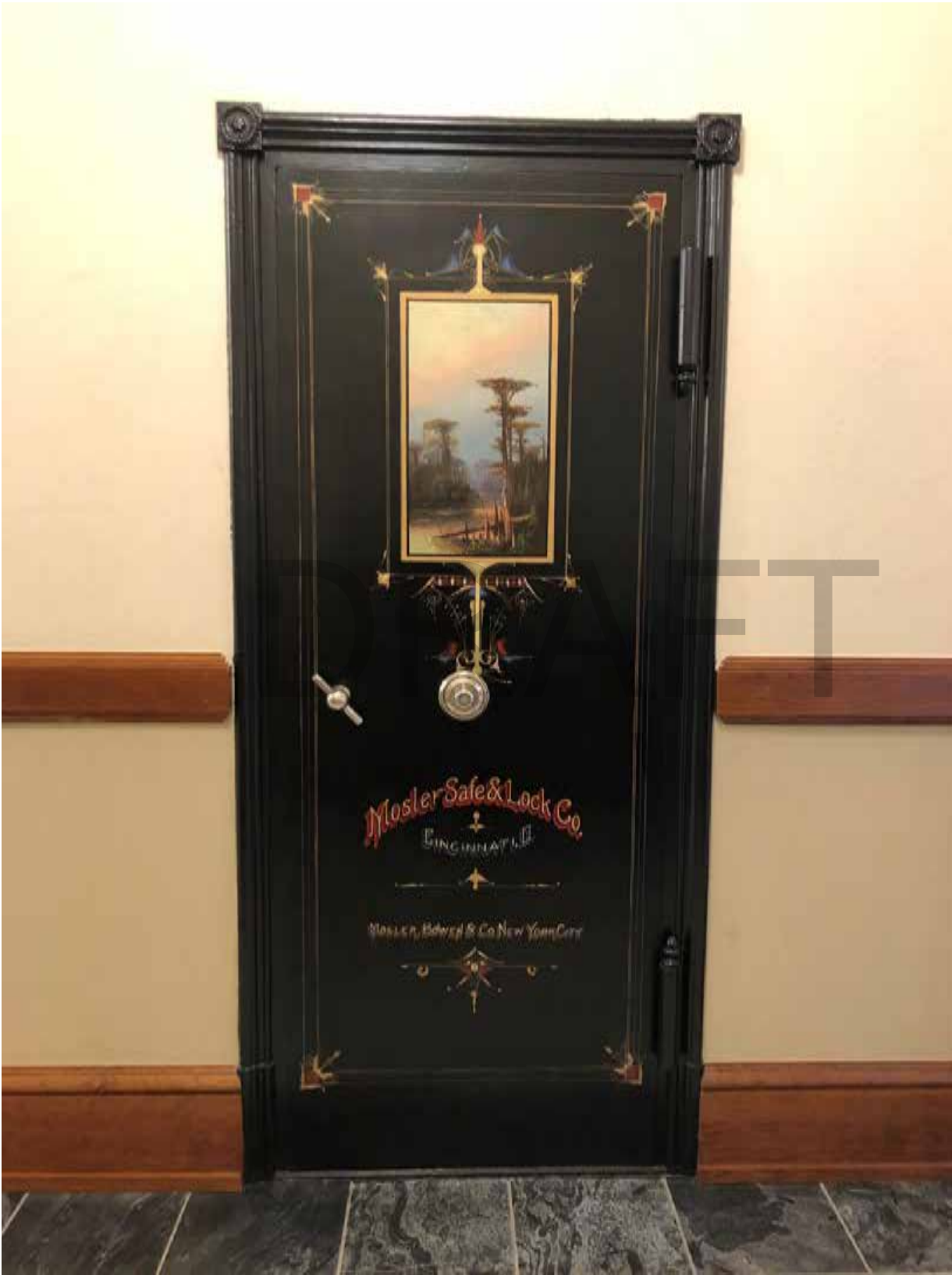
Photo 43 of 55: Detail of historic Mosler Safe & Lock Co. vault on the basement level. May 2021.
