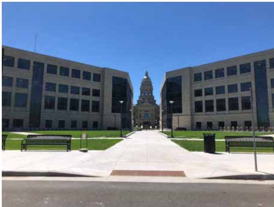
Photo 3 of 55: View of north Capitol entrance from 26th Street, looking through remodeled Herschler Building. A four-story atrium was removed from the Herschler Building to restore the view to the Capitol. Camera facing south. May 2021.
