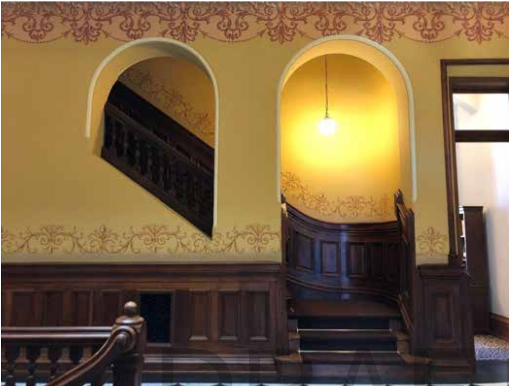
Photo 28 of 55: Enclosed second-floor stairwell on north wall leading to third floor. Camera facing north. May 2021.
