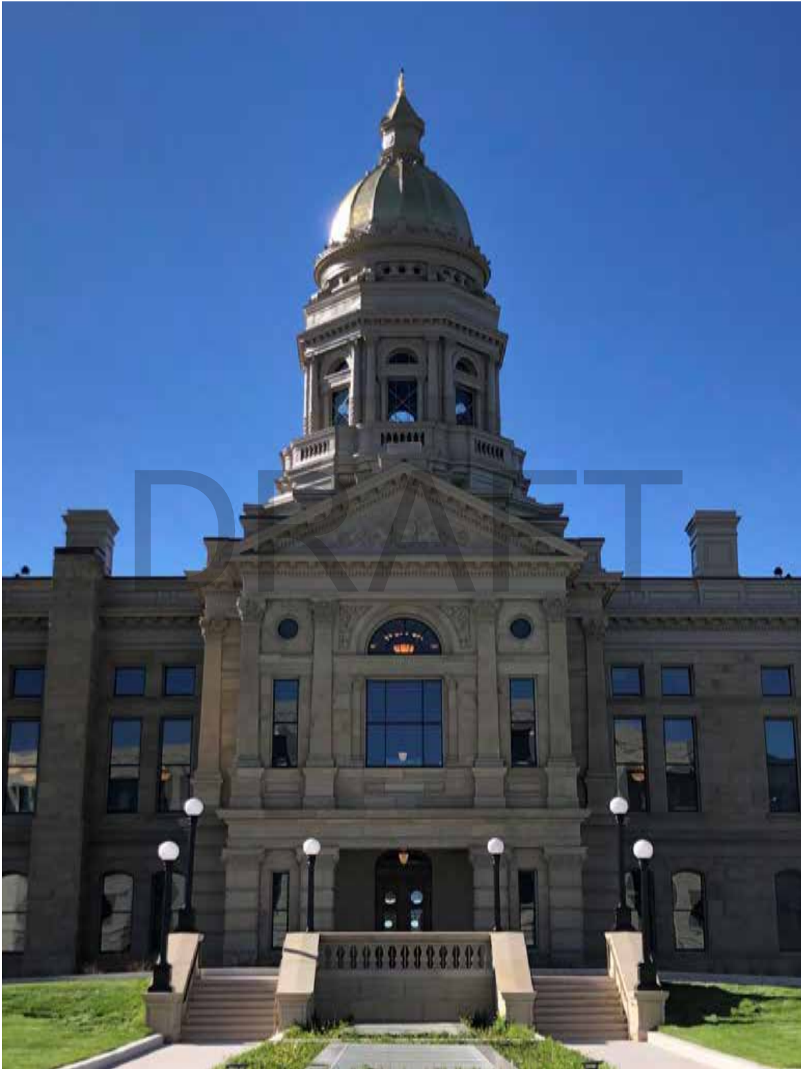
Photo 12 of 55: North side, monumental entrance pavilion and monumental stairs constructed in 1919. Camera facing south. May 2021.
