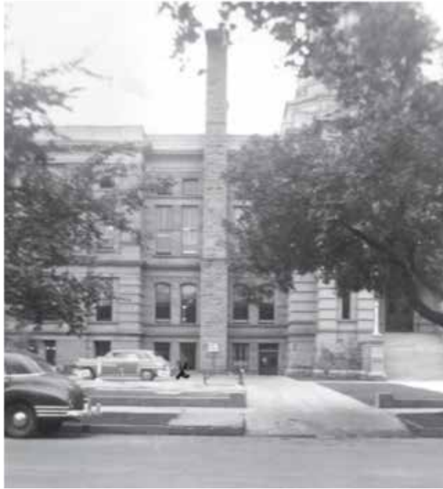
Figure 33: Capitol, north side ca. 1940s, after removal of existing north chimneys and construction of new chimney east of the north entrance. (Wyoming State Archives/P2006-26/052)
