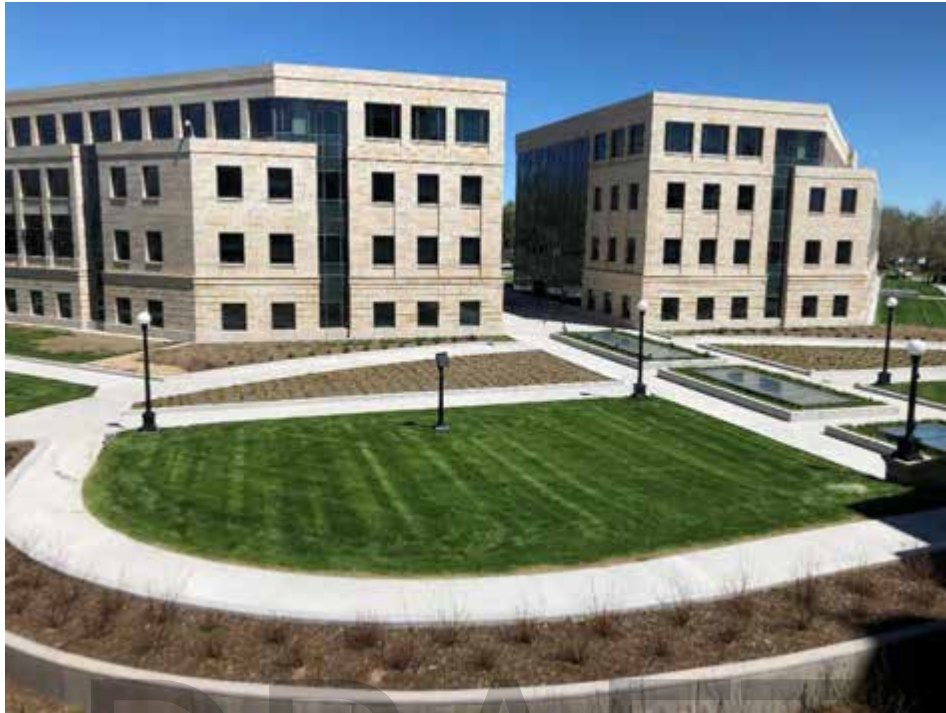
Photo 52 of 55: North lawn and Herschler Building, Capitol Extension skylights at right. May 2021.
