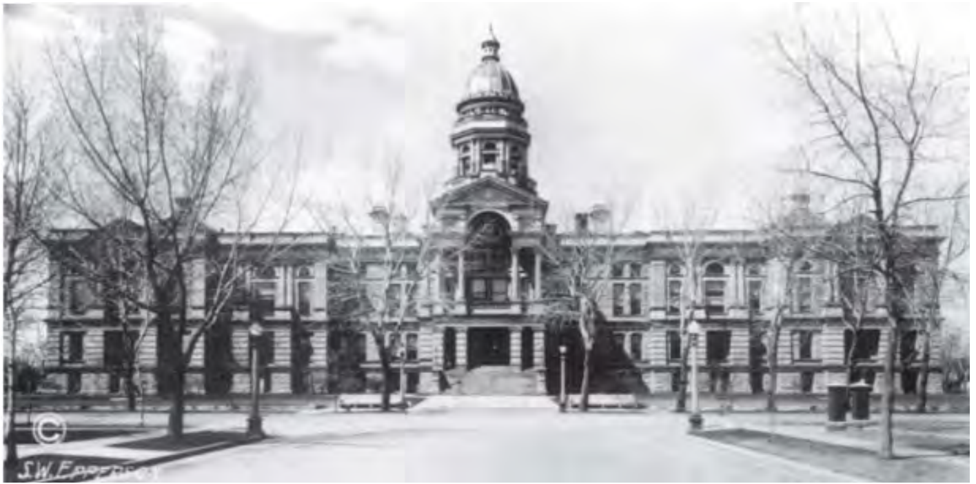
Figure 23: Capitol, south side, ca. 1920s after completion of the first landscape renovation. Photograph by Silas W. Epperson. (Wyoming State Capitol Renovation & Restoration Level I Reconnaissance & Level II Feasibility Study, 2013-2014/Wyoming State Archives)
