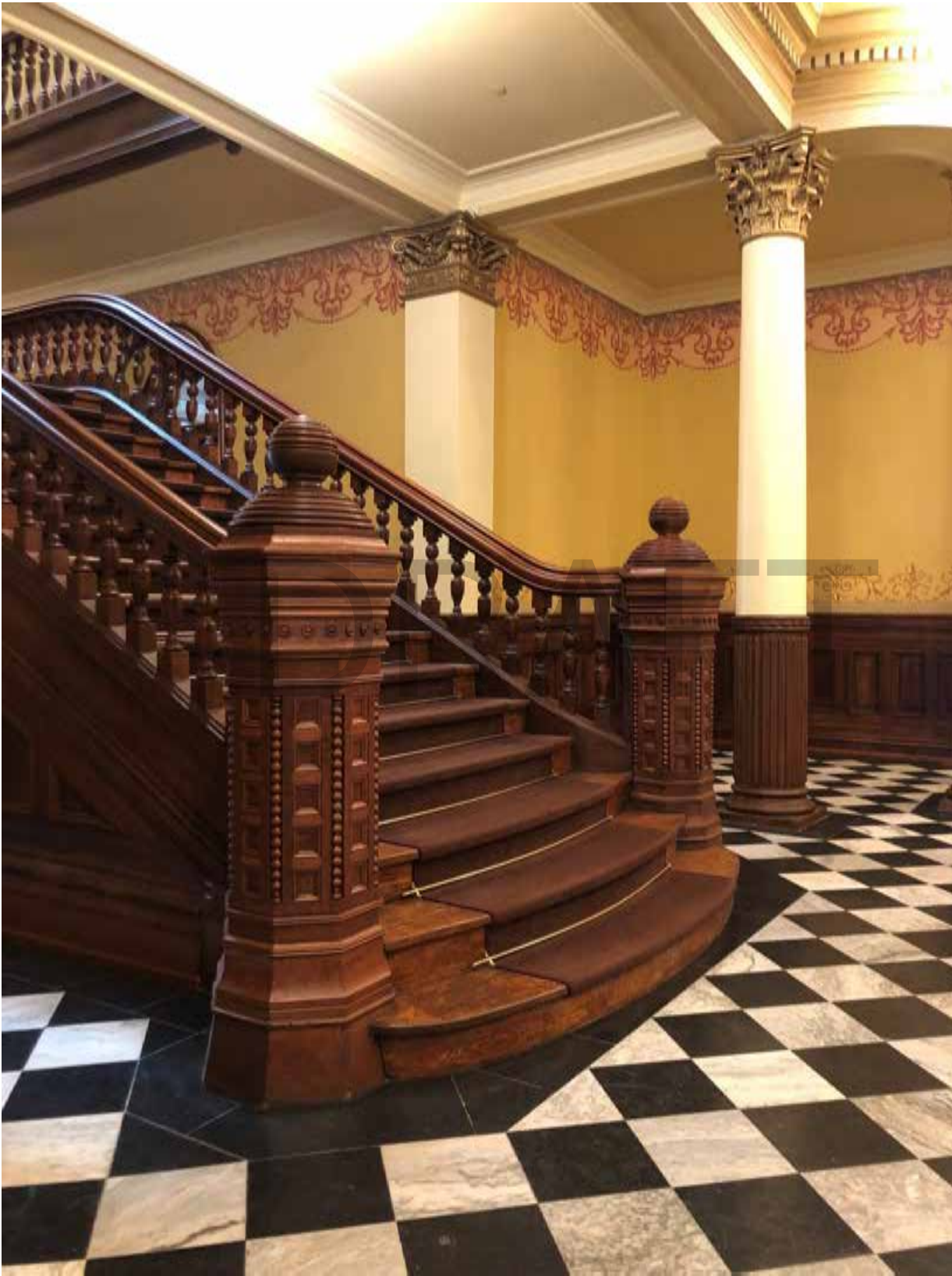
Photo 18 of 55: Detail of monumental staircase, cast iron column, wall treatment and marble flooring. Camera facing southeast. May 2021.
