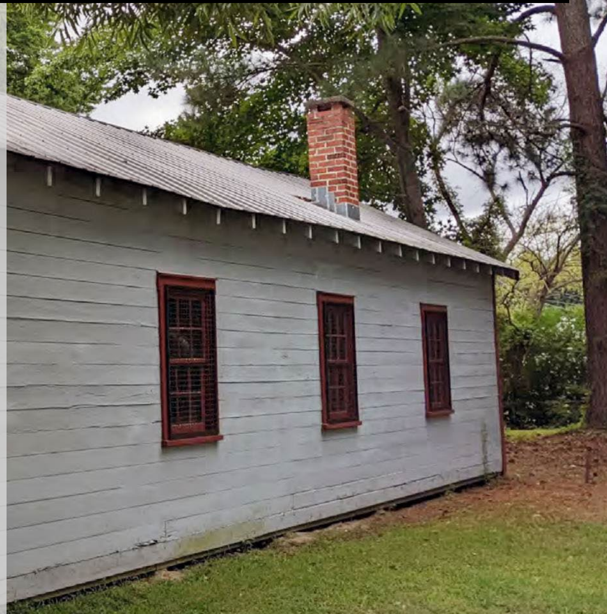
Samuel D. Outlaw Blacksmith Shop (VA), built c. 1927, listed 2023.
