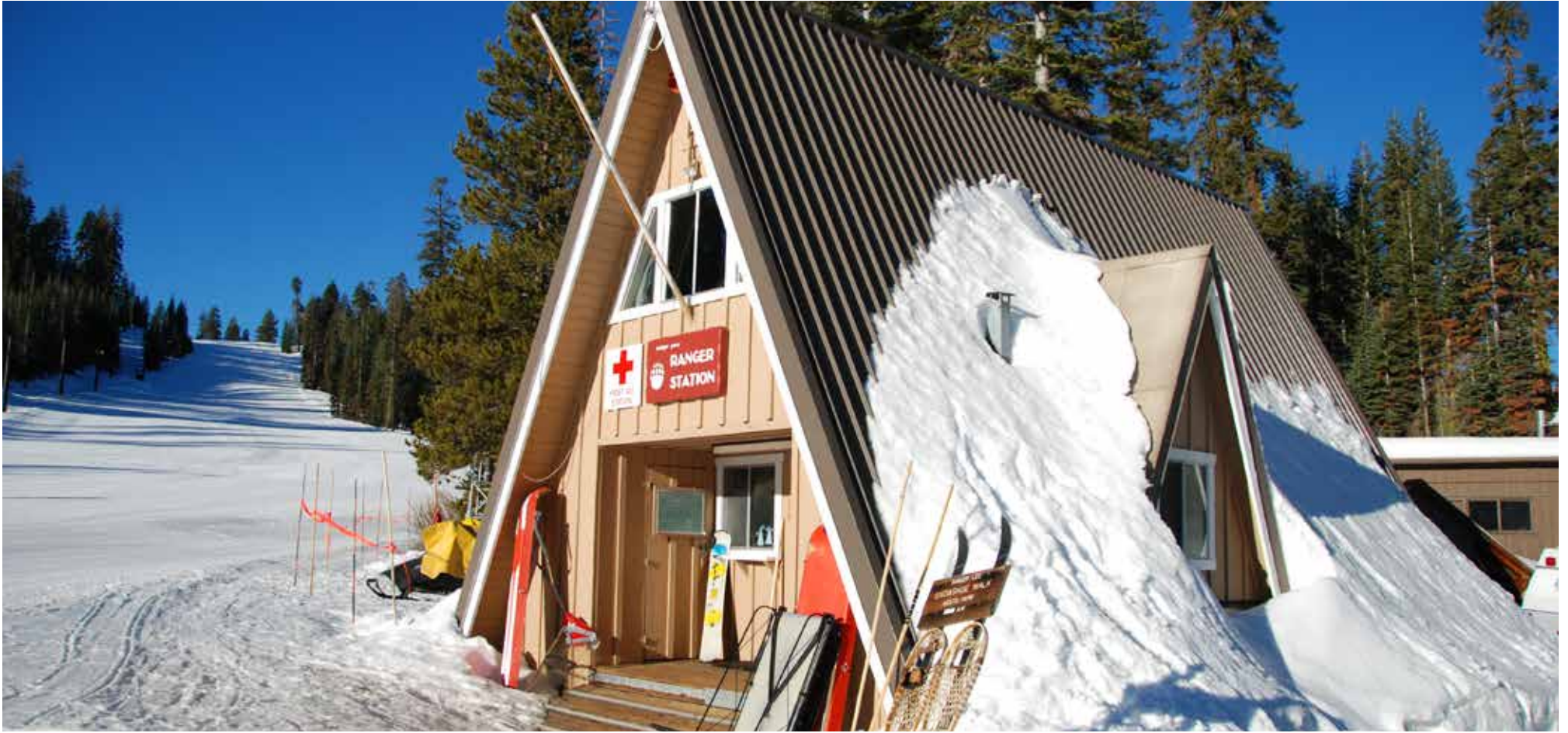
The Badger Pass Ranger Station A-frame. NPS Photo
